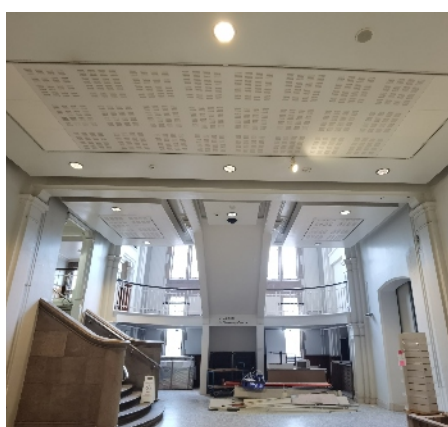
Photographs of the existing conditions within the main hall
