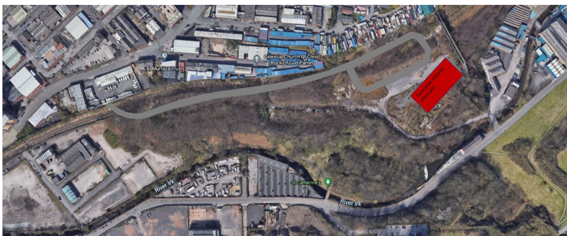
Stage 4 Road construction complete, stockpiles tidied and all machinery removed form site.
