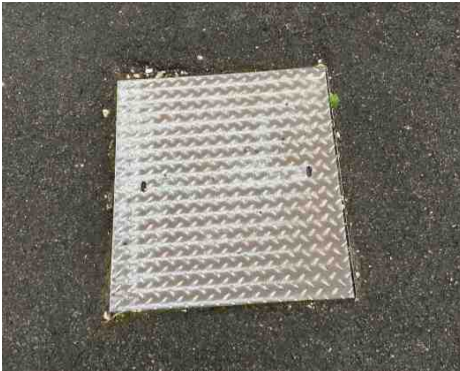
Photograph 4: A manhole cover located on site adjacent to the eastern single- storey building's public entrance.
