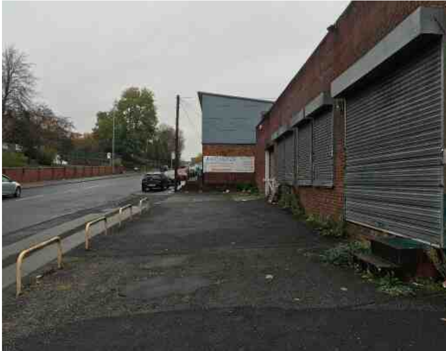
Photograph 1: View of the proposed access road towards the northwestern boundary which connects to Waterloo Road.
