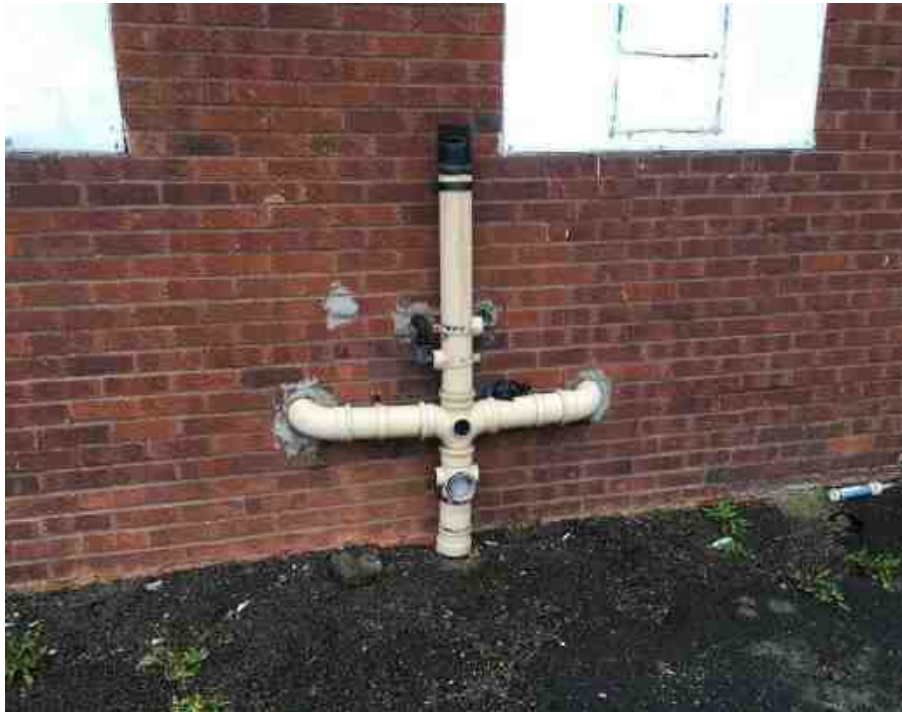
Photograph 2: A drainage pipe located on the current property's eastern side which suggests there is an established connection to the combined sewer adjacent to the site.
