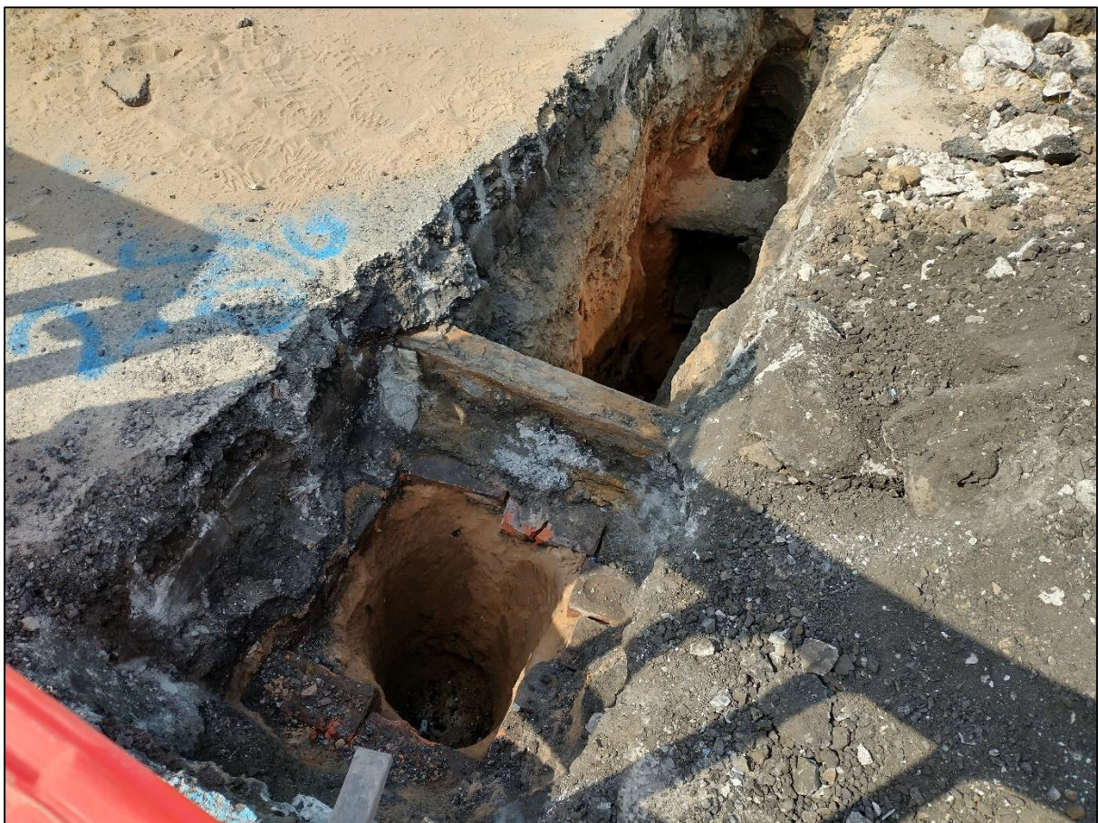
Plate 1: Tram track visible within a service trench, looking west
