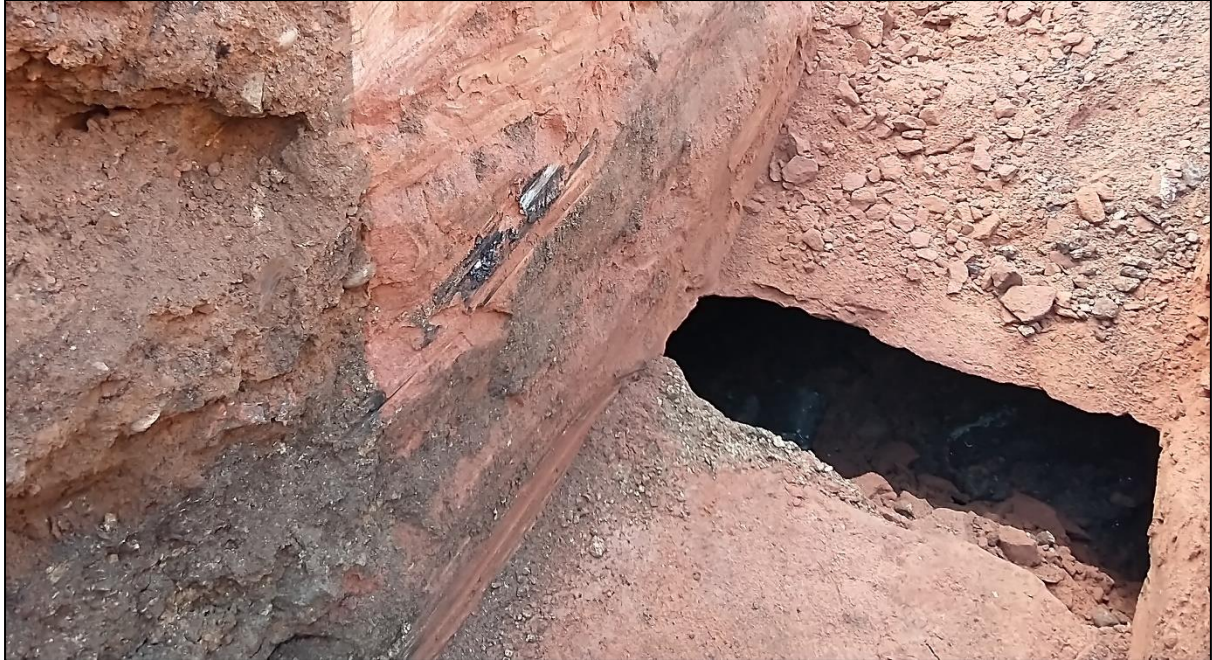
Plate 2: Natural fissure within the bedrock, looking north
