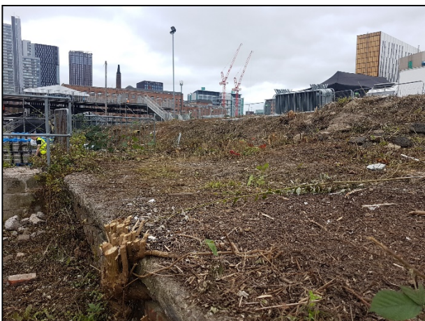
Photo 4 Area of cut vegetation projecting from western boundary
