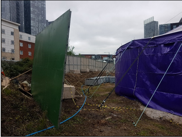
Photo 2 South-west boundary showing cut vegetation
