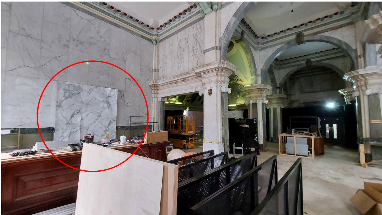
Plate 7: The fake marble panel covering area of former doorway.
