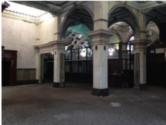
Figure 1. View through to the Clerks Hall from the south-east corner of the building (on plan) demonstrates the impact the former relocated counter and security screen had on
