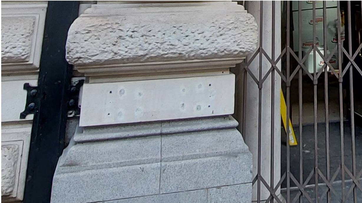
Plate 9: The numerous drill holes where the signage will affix.
