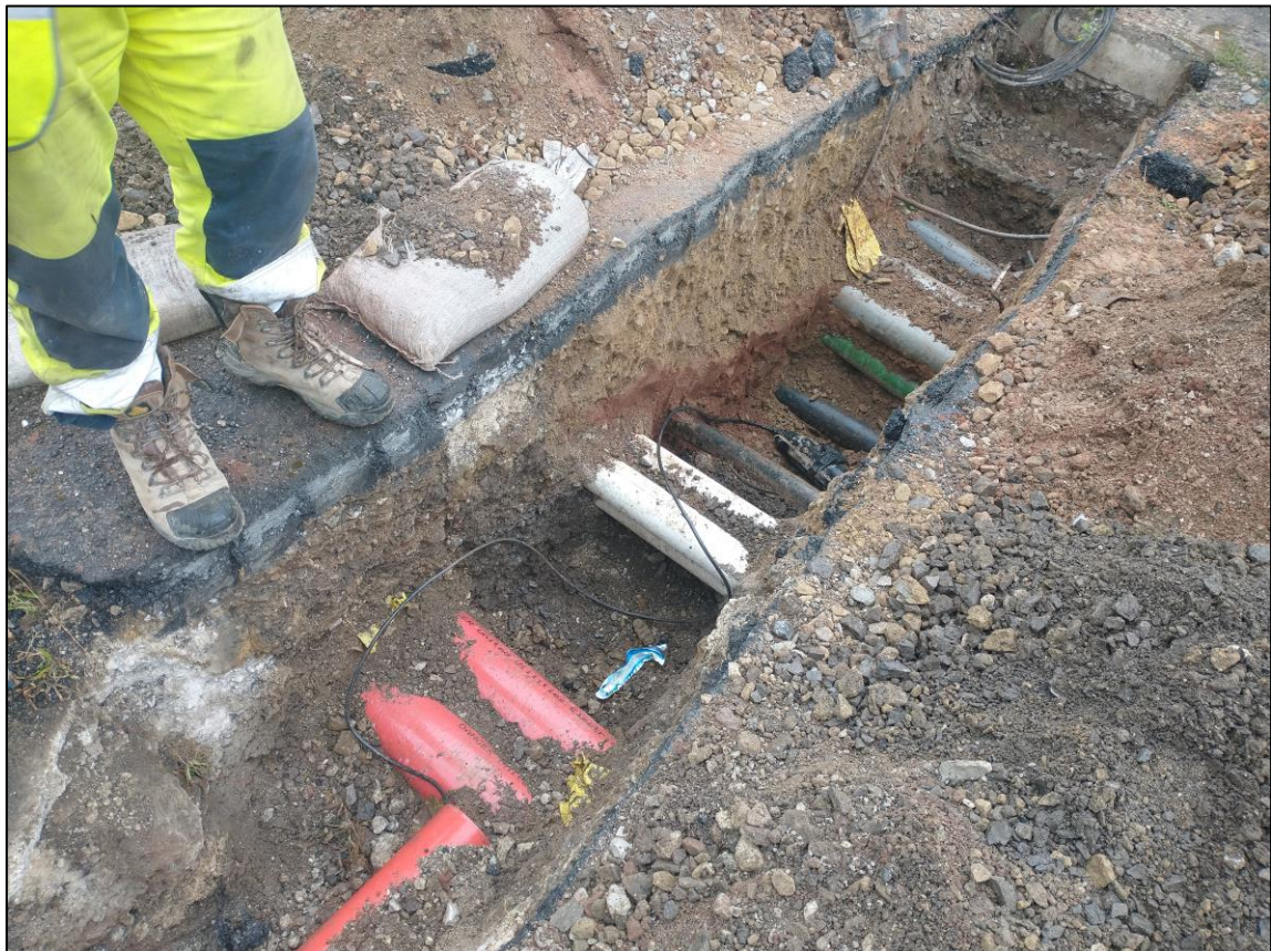
Plate 8: Services and drainage below the pavement
