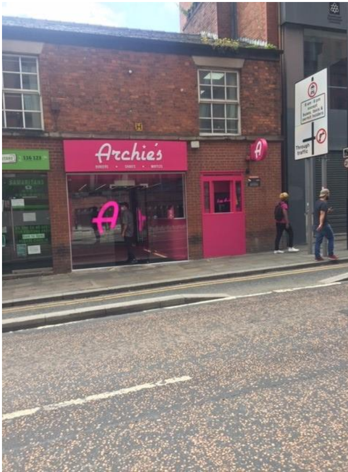
FIGURE 2 FRONT OF 72 OXFORD STREET ON 16TH JULY 2021
