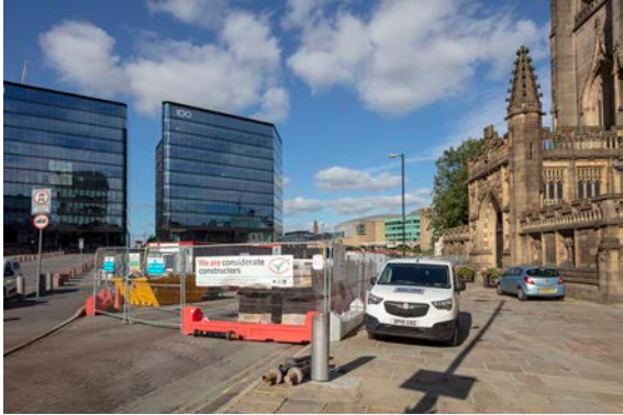
VP 03 - Junction of Victoria Street with Cathedral Yard
