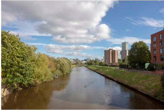
VP 06 - Broughton Road Bridge
