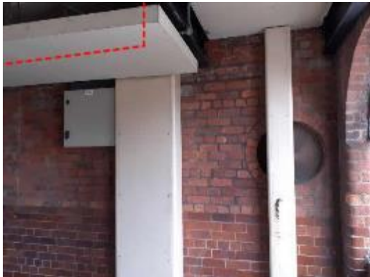
Picture showing cable route.
