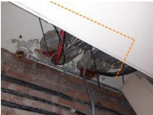
Picture showing power cable route.
