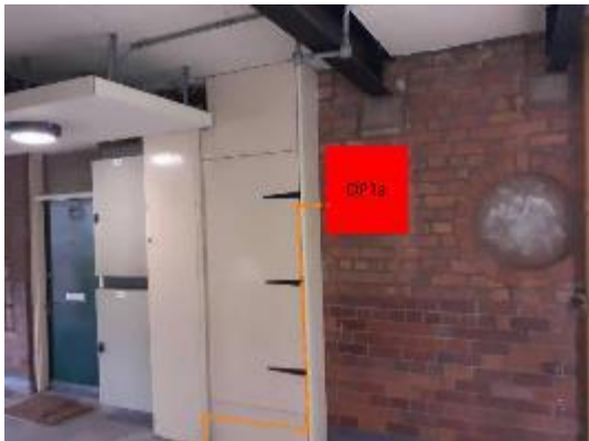
Picture showing power cable route.
