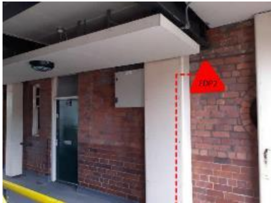
Picture showing cable route.
