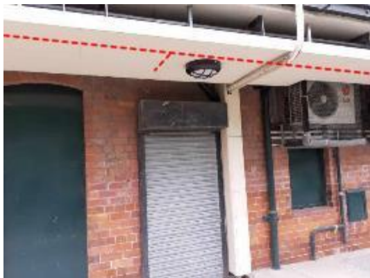
Picture of the Business unit on Ground floor.
