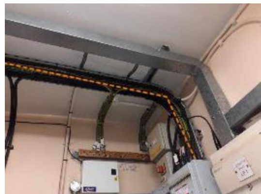
Picture showing power cable route.
