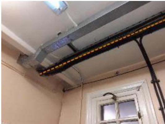
Picture showing power cable route.
