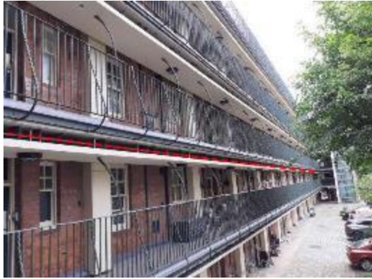
Picture showing cable route.
