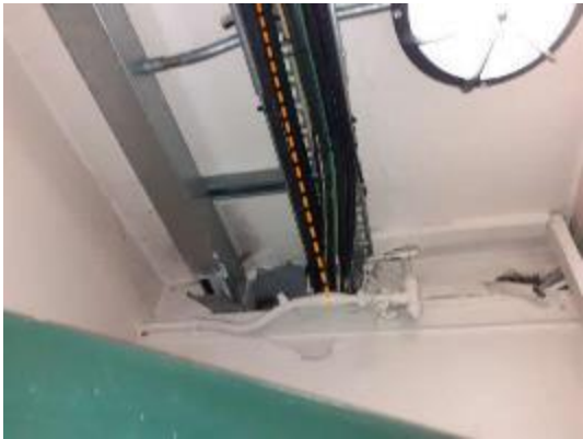
Picture showing power cable route.
