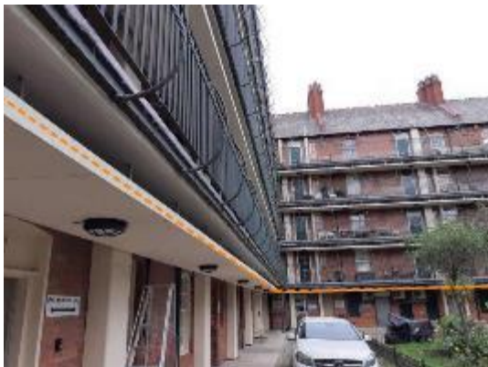
Picture showing power cable route.
