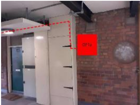
Picture showing cable route.
