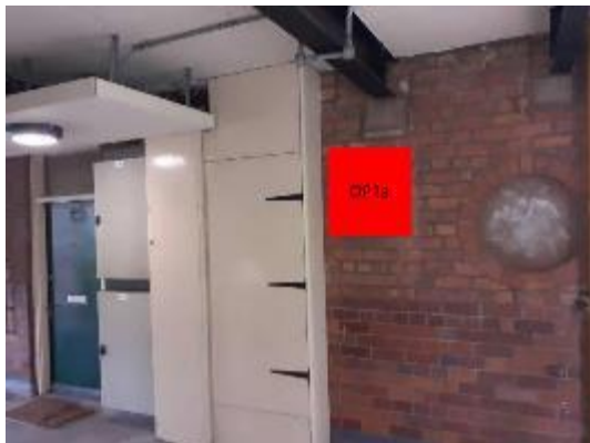
Picture showing the Cabinet location next to 20A.
