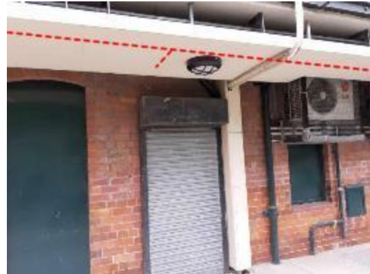
Picture showing connection for business units.
