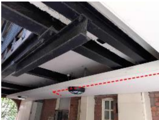
Picture of cable route at of the run.
