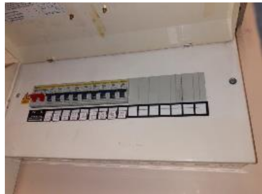
Picture showing spares in DB.
