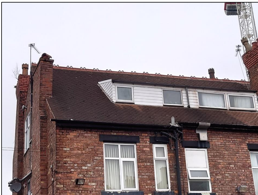
Photograph 3 showing the roof at the rear of the property
