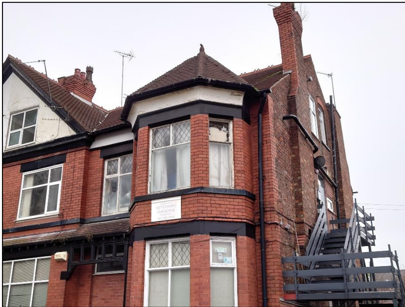
Photograph 1 showing the front elevation of the building
