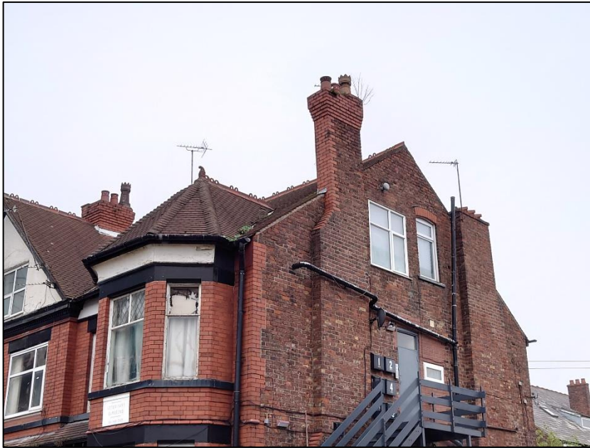
Photograph 4 showing the roofing at the front of the property
