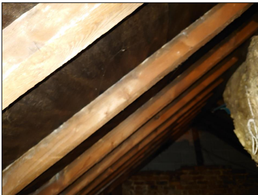
Photograph 5 showing the roof joists
