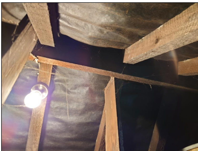
Photograph 6 showing the roof void
