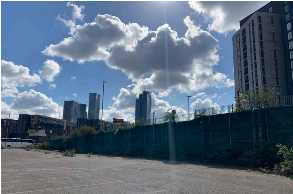
View looking south east along the retaining wall of Regent Road
