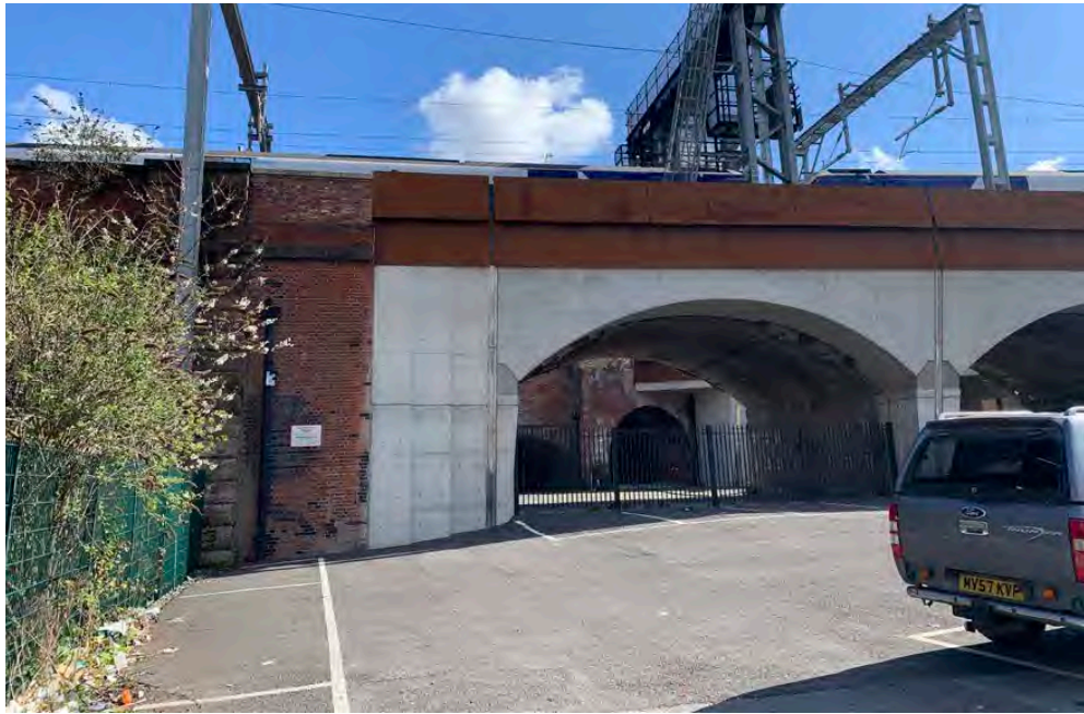
The existing character of the site is strongly influenced by the railway line, railway steel stanchions and the arches. The structure is a listed.
