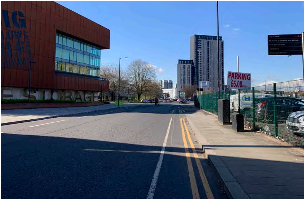
View along Water Street with Site C to the right of the photo and the storage unit to the left. Recent footway improvements along the storage unit footway. The footway adjacent to the site is partial paved in natural stone
