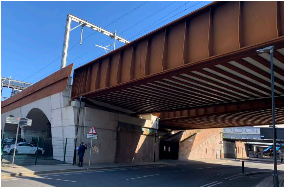
The character is bold and industrial, with corten, concrete, brick and steel. The recently clad bridge brings the bridge into further focus
