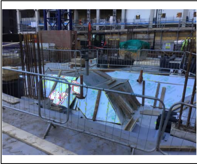
Overview of Gridline 5-7 being
