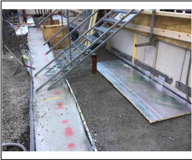
Membrane to connect ring beam
