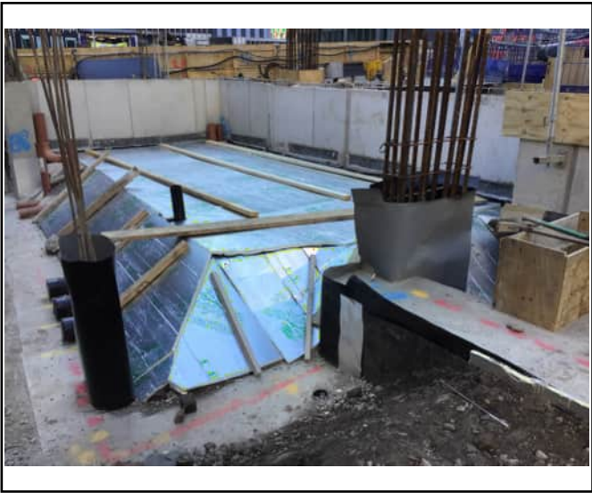
Next section to install in insulation
