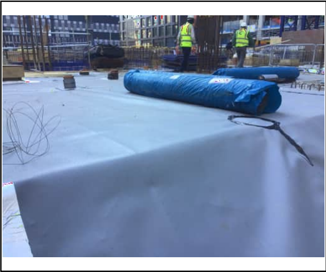
Overview of verified section
