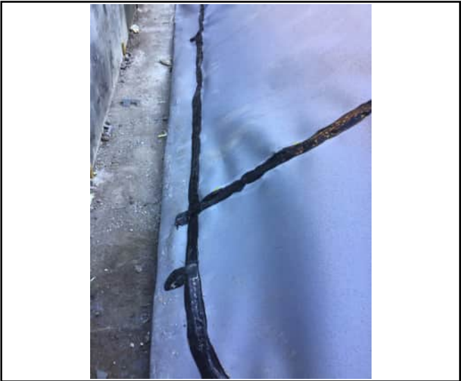
Extrusion welds on the slope
