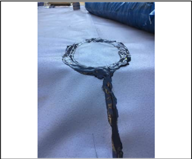
Extrusion welds
