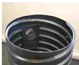
Insert the back plate into the rodding eye of the gully
