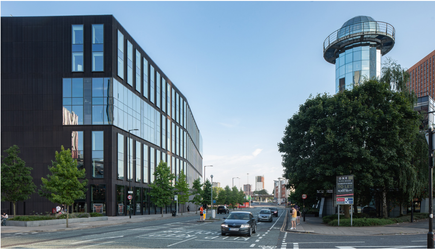
View from Medlock Street looking south
