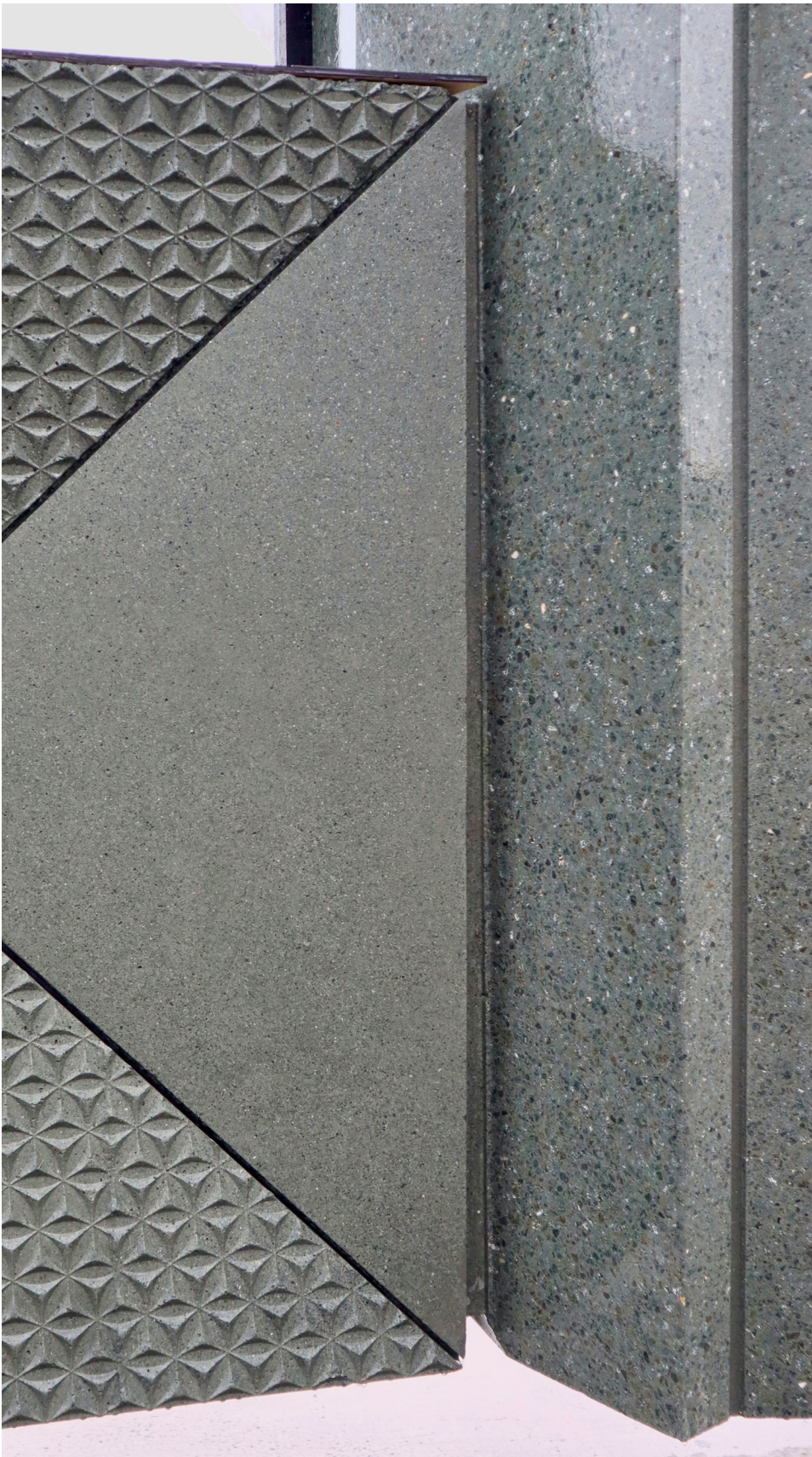
Detail showing polished vertical and detail with horizontal panel
