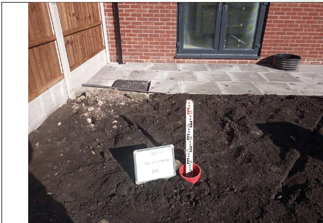
Photograph 2: Validation of Garden Capping Thickness
