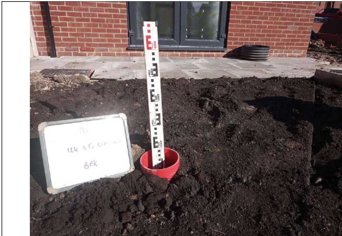
Photograph 1: Validation of Garden Capping Thickness
