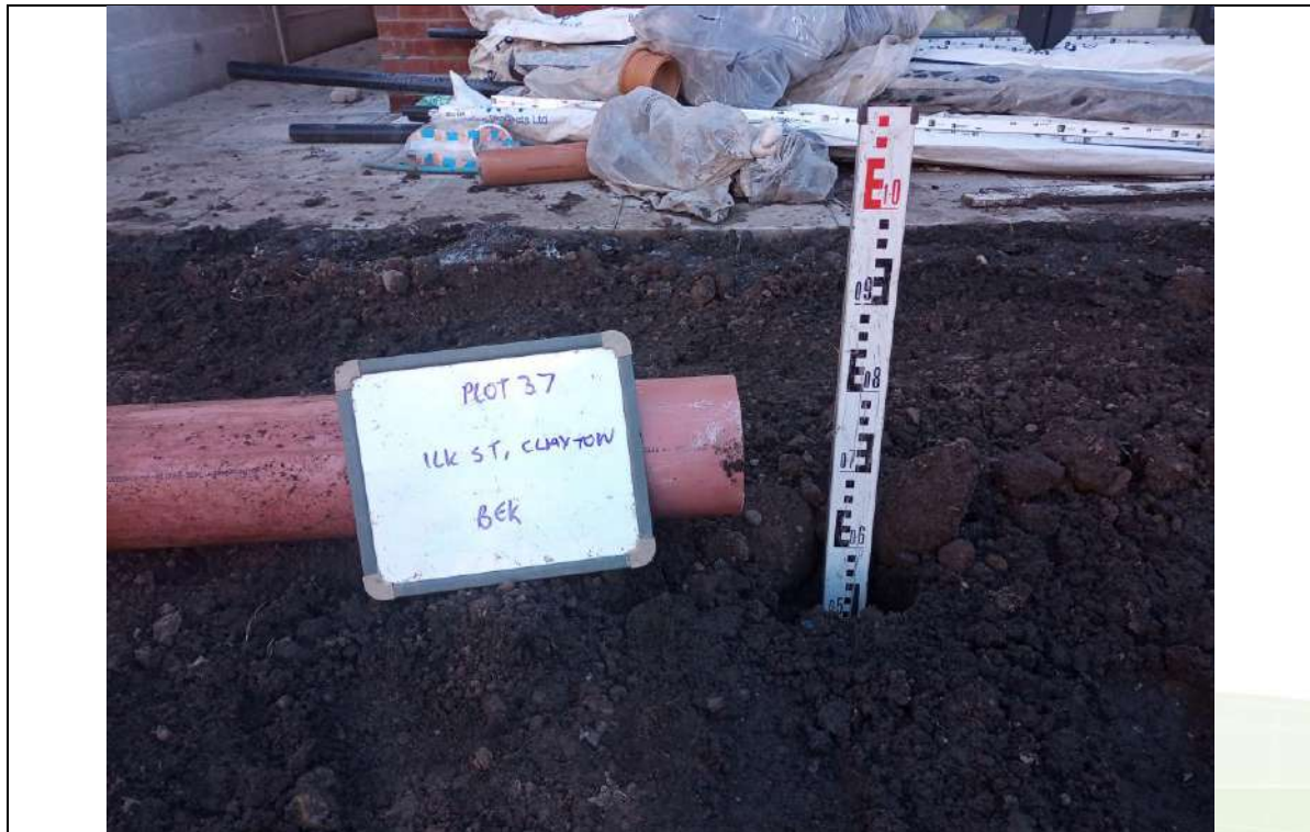
Photograph 1: Validation of Garden Capping Thickness
