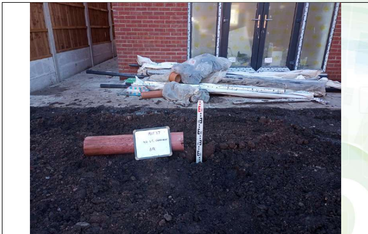
Photograph 2: Validation of Garden Capping Thickness
