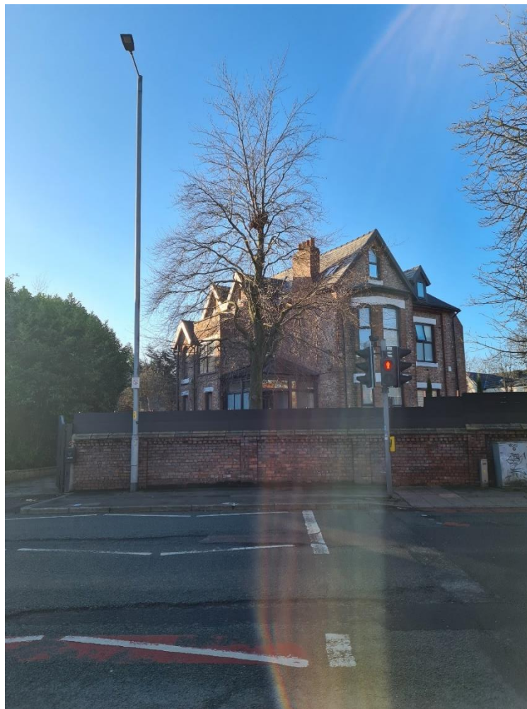
Figure 5.2: View looking south towards the application site from
