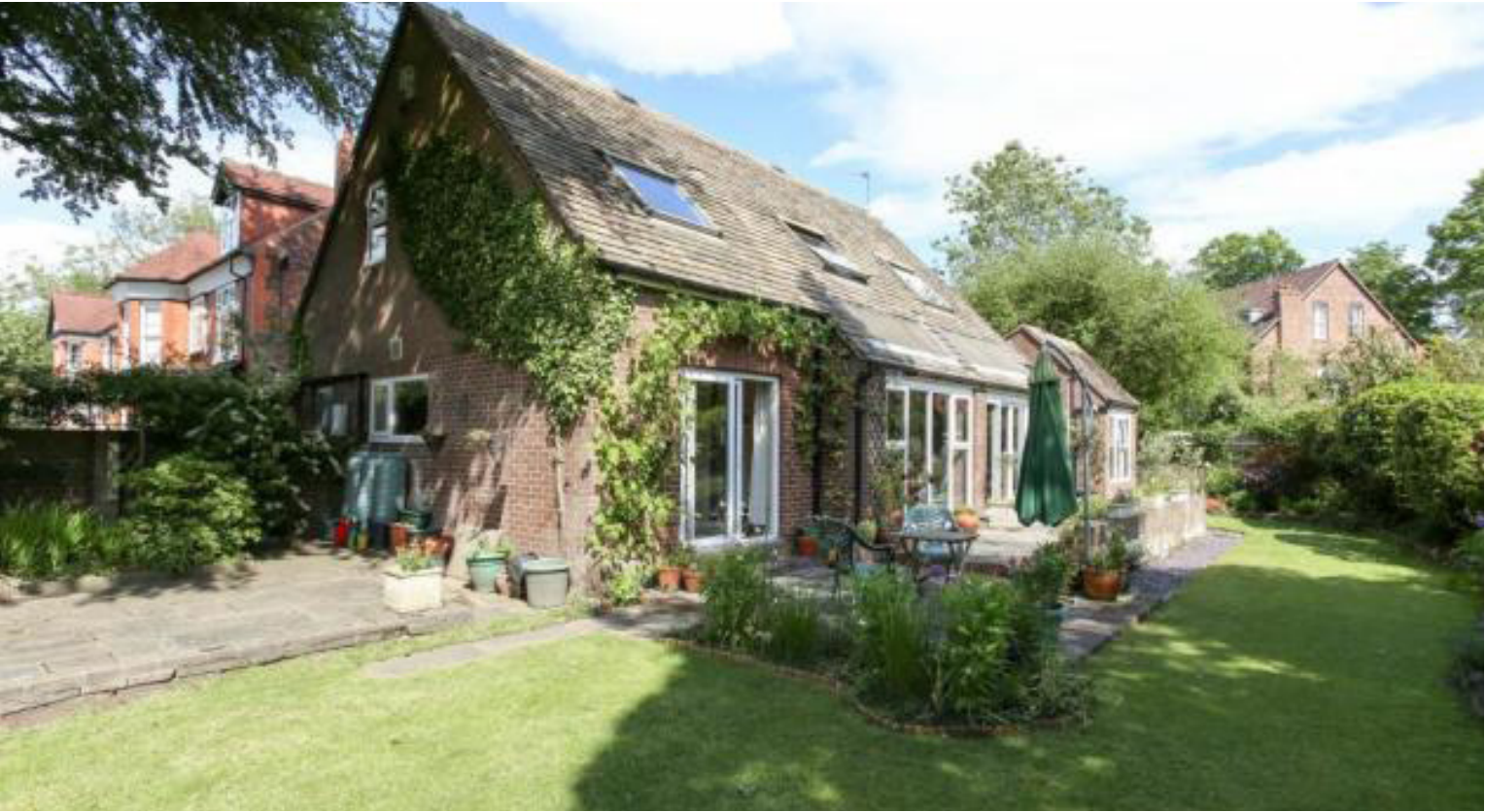
Gable end elevation of 3 Winster Avenue
