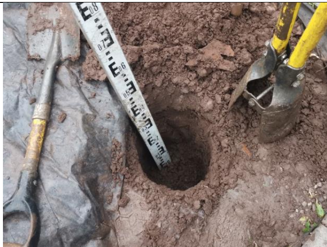
Hand Dug Pit 05: Overview of excavation
