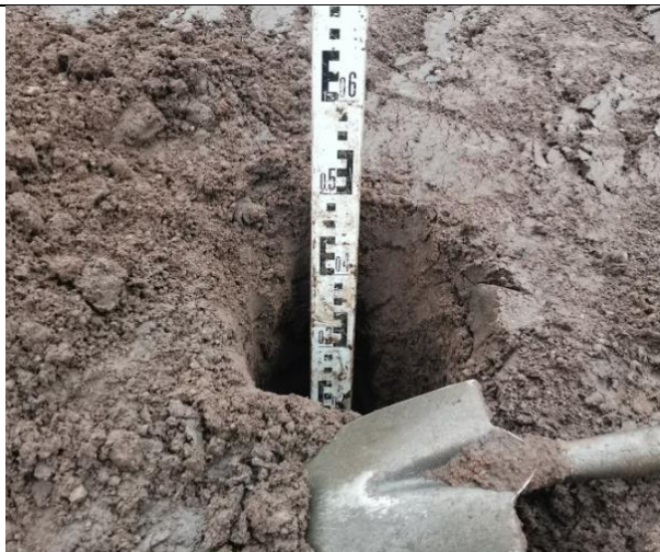
Hand Dug Pit 07: Overview of excavation
