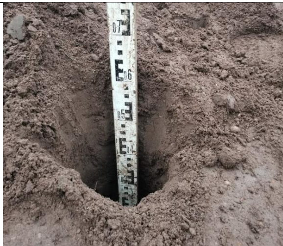
Hand Dug Pit 08: Overview of excavation
