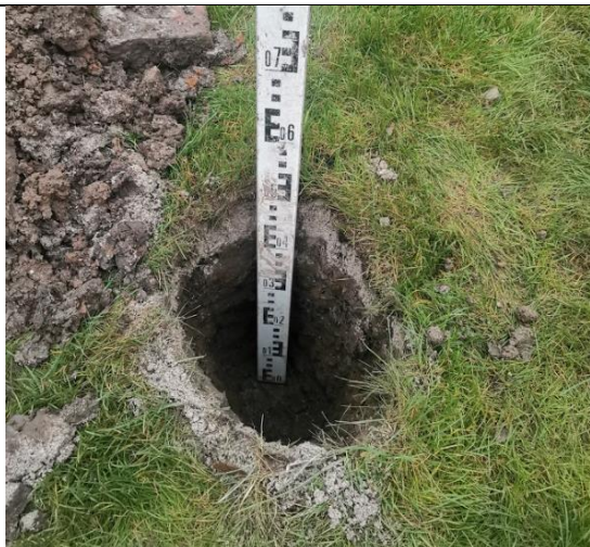
Hand Dug Pit 01: Overview of excavation
