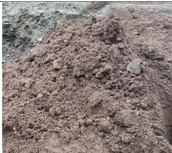
Hand Dug Pit 08: Overview of excavated soils
