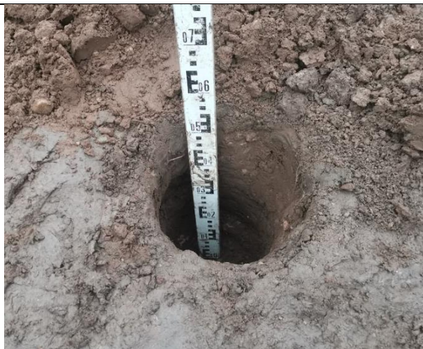
Hand Dug Pit 04: Overview of excavation
