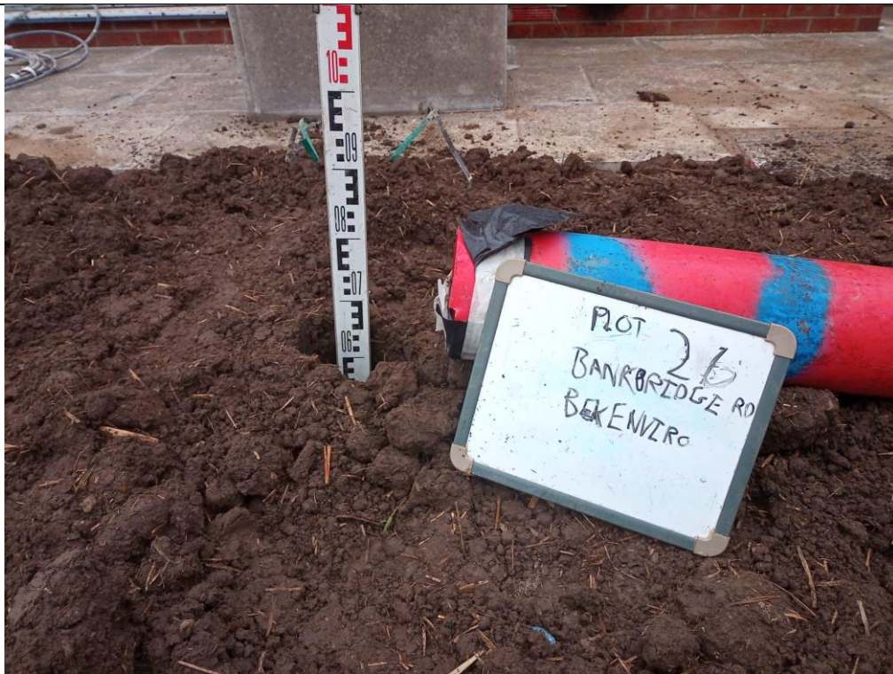
Photograph 1: Validation of Garden Capping Thickness
