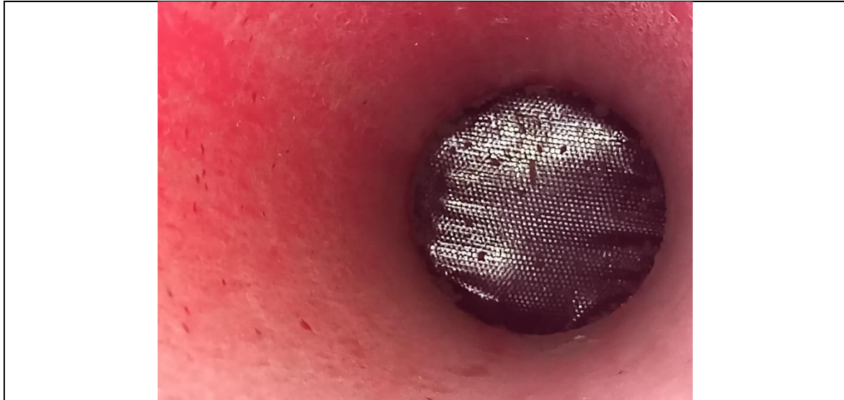
Photograph 3: Validation of Geotextile Membrane
