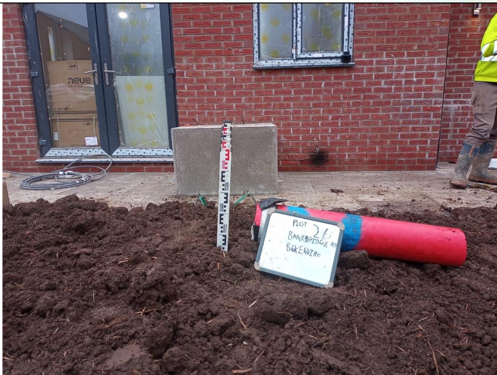
Photograph 2: Validation of Garden Capping Thickness
