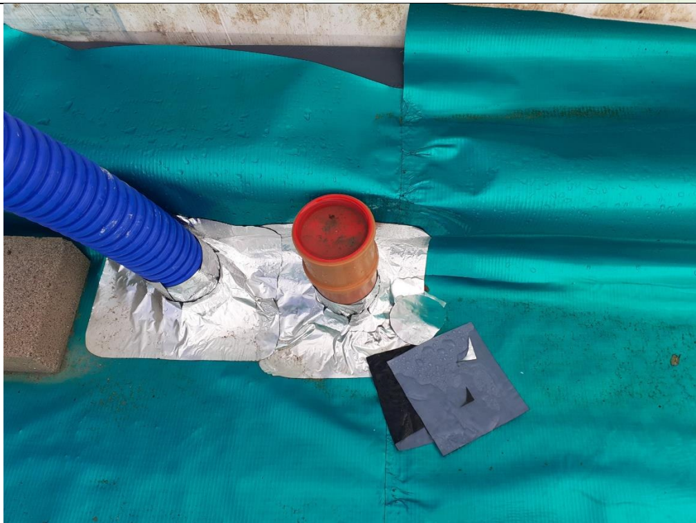
Photograph 6: Validation of Gas Membrane Installation
