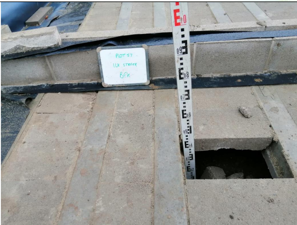
Photograph 4: Validation of Sub-Floor Void Space (min 150 mm)
