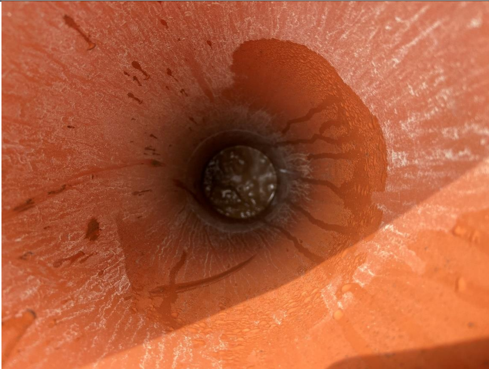
Photograph 3: Validation of Geotextile Membrane
