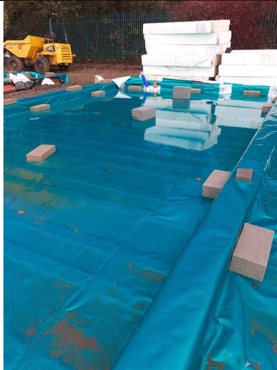
Photograph 5: Validation of Gas Membrane Installation
