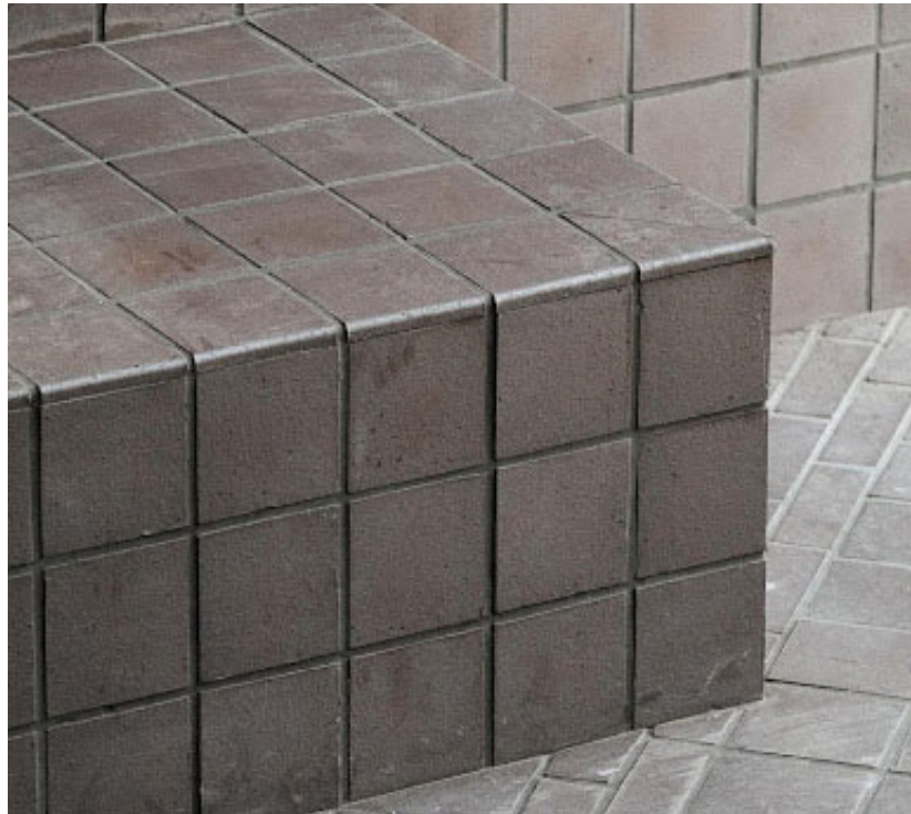
2.5 Quarry tiles: floor, low level wall & seat base tiling. Specification: Ketley Brick Brown Brindle Quarry tiles
