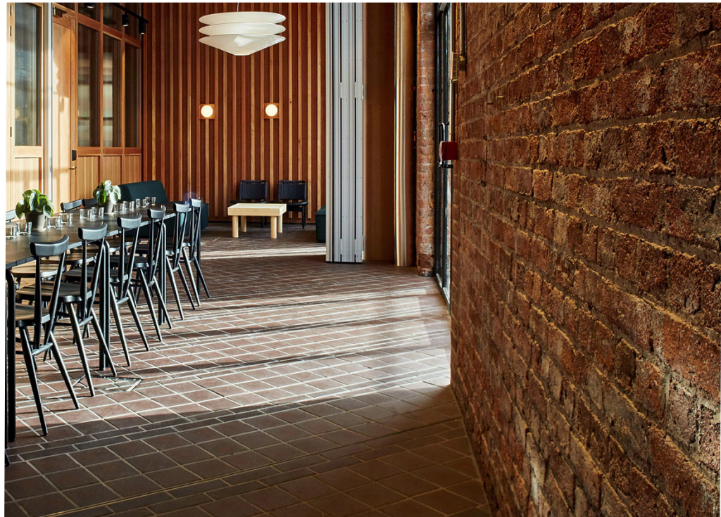
2.5 Quarry tiles: floor, low level wall & seat base tiling. Specification: Ketley Brick Brown Brindle Quarry tiles
