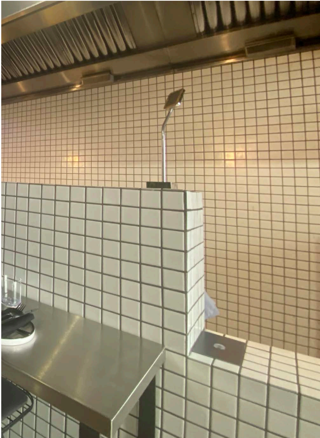
2.6 Wall tiles: high level only. Light grey square matt ceramic wall tiles These wall tiles are used at high level and form a neat strip above the mirror panels to new walls (only).
