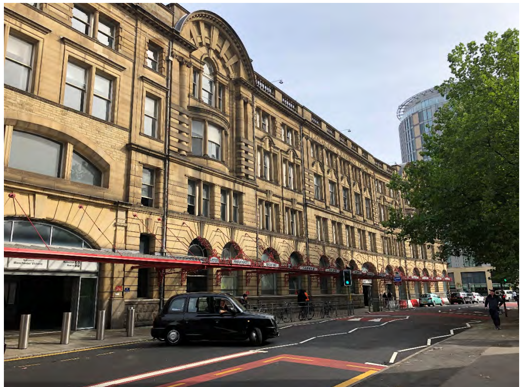
Plate 11 Principal (southwest) elevation of the Grade II listed Victoria Railway Station. Image taken from the southwestern flank of Victoria Station Approach.
