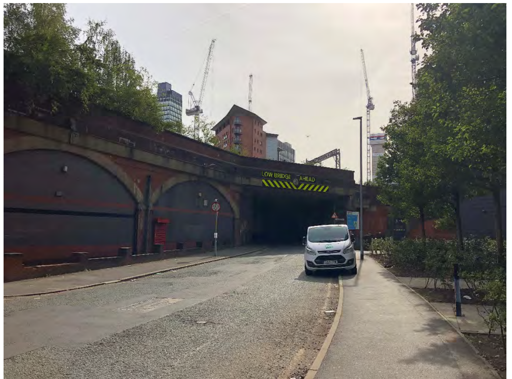
Plate 6 View southwest along Red Bank illustrating the visual severance between the Grade II listed Victoria Station which is located c. 298 metres from this location (arrowed) and the immediate environs of the subject site.
