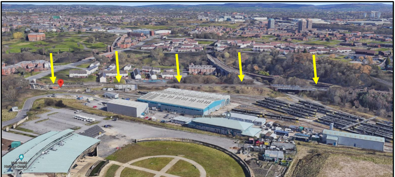
Figure 5.9: Visible Queens Road metro line section from depot
