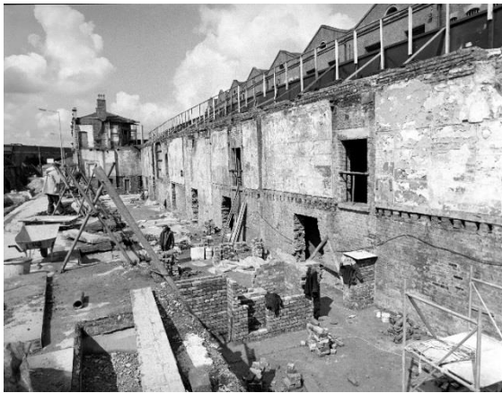
Figure 3 The Station Building c.1985 showing the extent of the reconstruction
