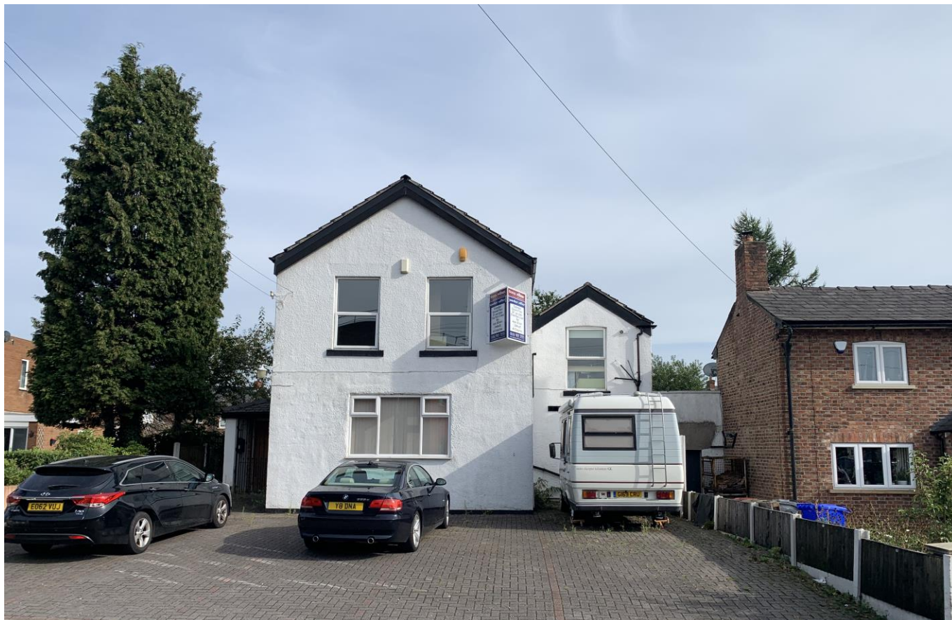
Photograph 1 Front Elevation as viewed from Moor End Road
