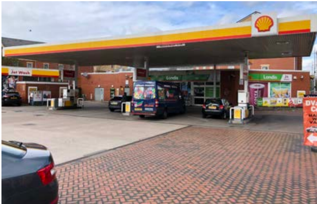
Plate 3 View of the existing forecourt and shop building looking north, jet wash on left.
