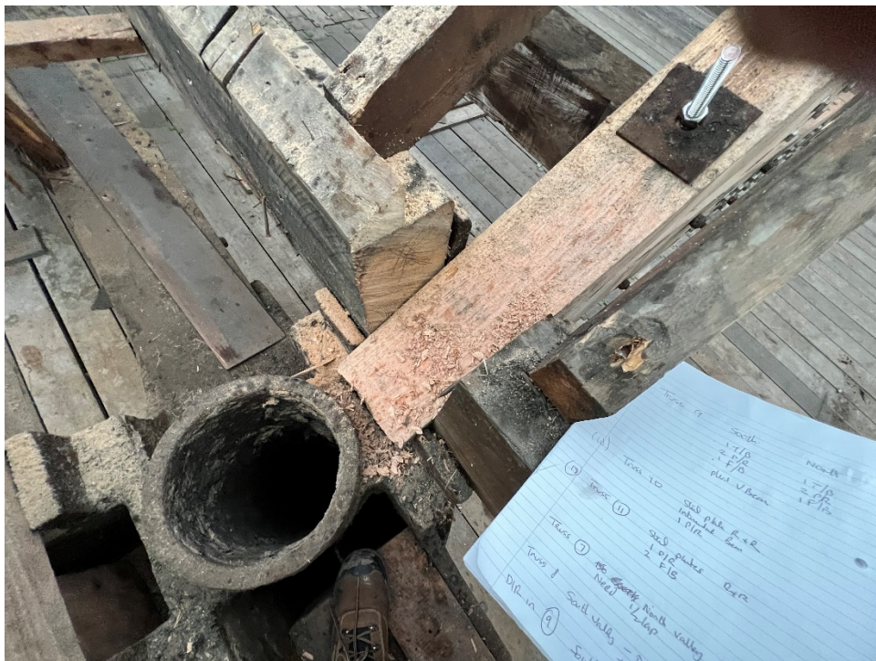
Truss 12 Valley Beam South Side
