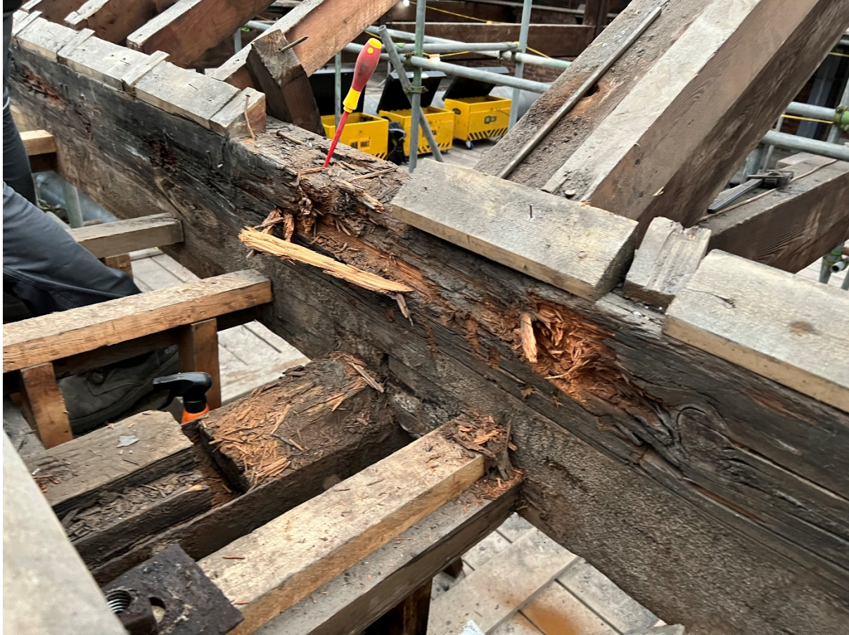
Trusses 12 to 13 Valley Beam North Side
