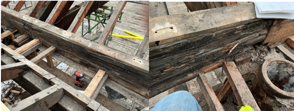
Trusses 12 to 13 Valley Beam South Side
