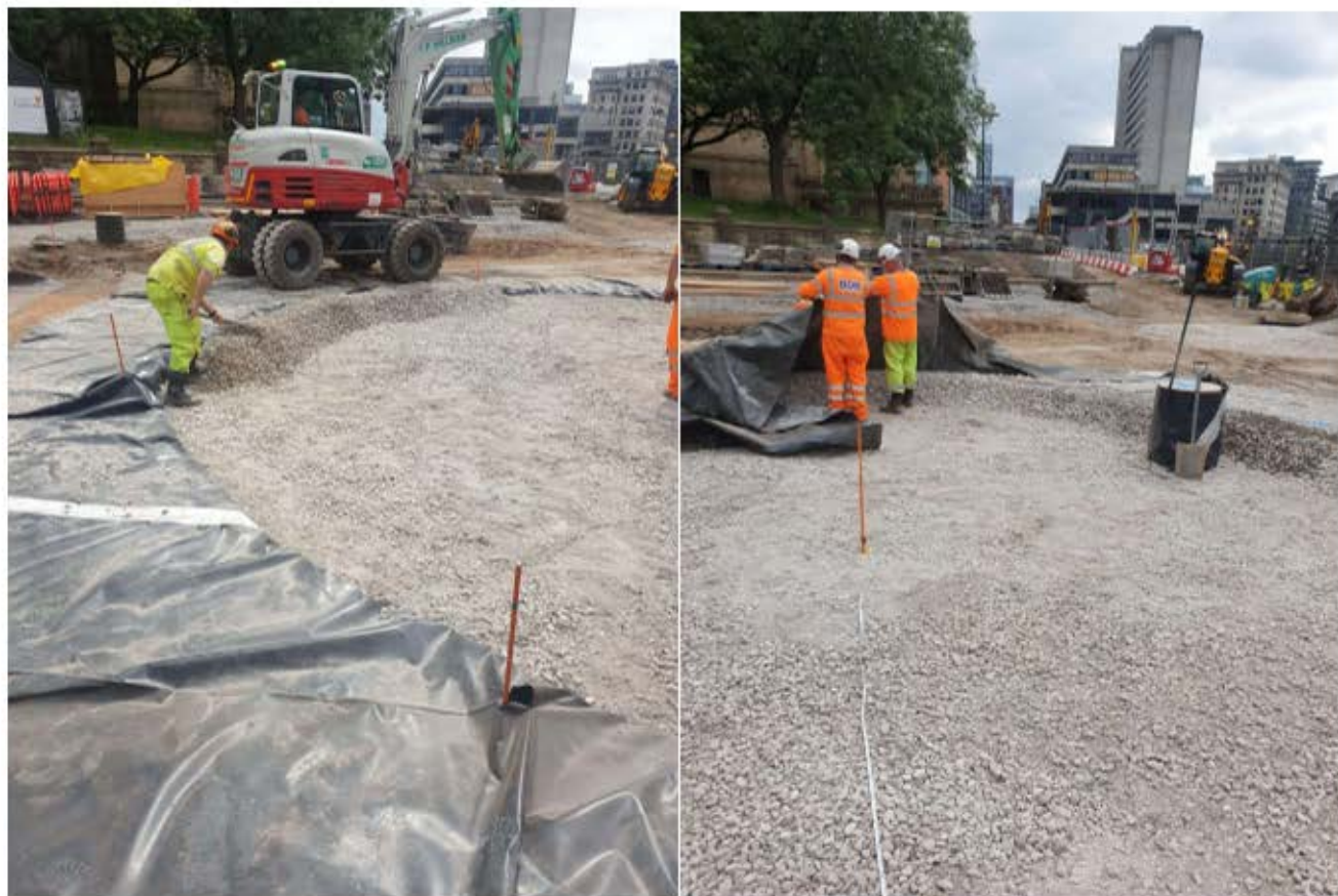
Raingarden blanket - Type 3 MOT to blanket and filter drain surround Left: Forming filter drain to perimeter of raingarden Right: Trimming impermeable membrane to edges of filter drain
