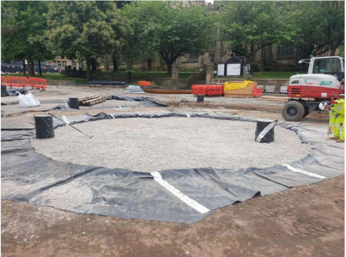
Raingarden to central Halo prior to permeable membrane installation
