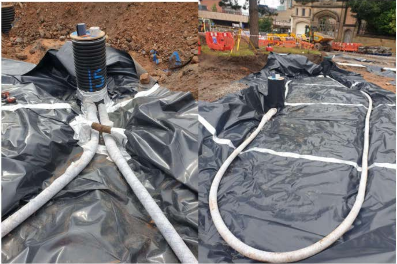
Filter drain installation. Filter drain pre-wrapped in permeable geotextile
