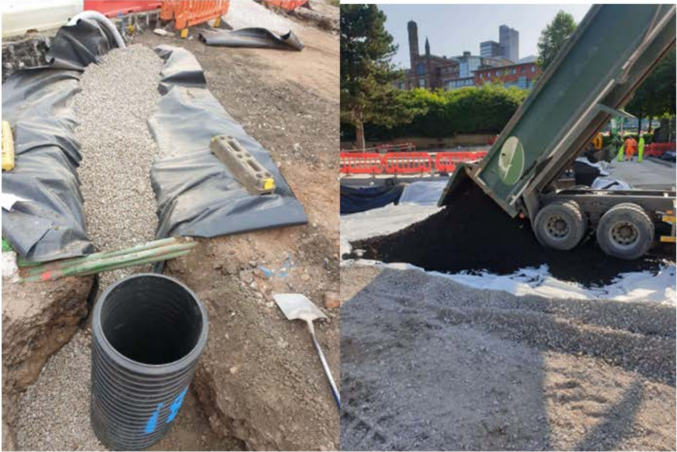
Filter Drain installation
