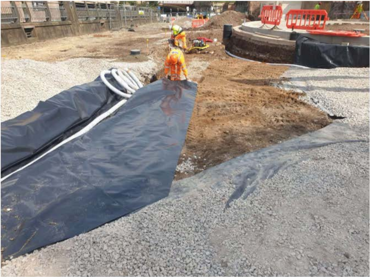
Impermeable membrane and filter drain installation
