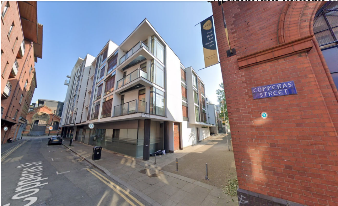
Figure 2: Parking space located on Copperas Street adjacent to the premises.
