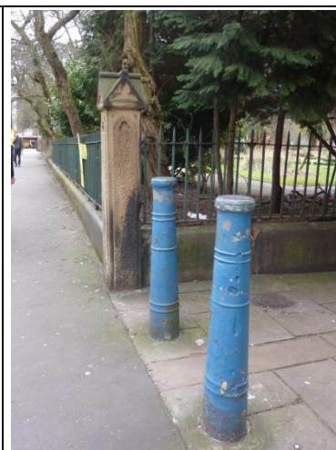
One set of the Listed Bollards next to St. John's Gardens
