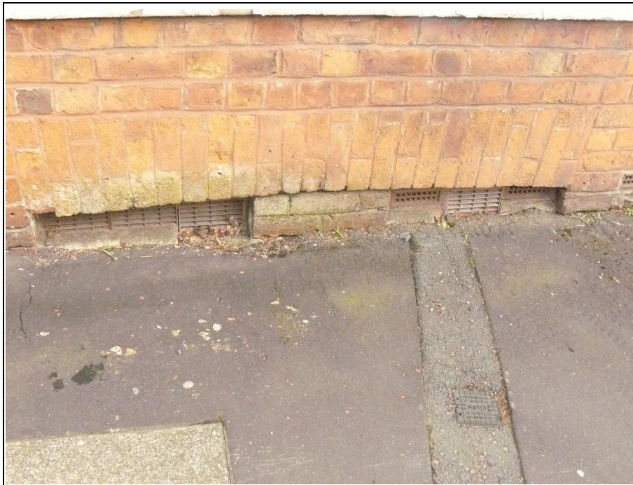
Ventilation to Cellar Rooms
