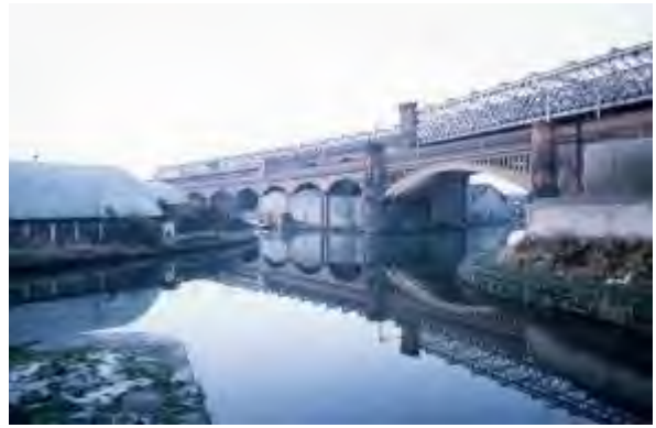
Figure 24: 1987- Looking west from the 92nd lock of the Bridgewater Canal, illustrating the dereliction of the area at this time.
