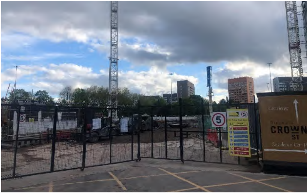
Figure 33: Looking west into the former Pryme Street, showing the groundworks being undertaken for the initial phase of the Crown Street Phase 2 development.
