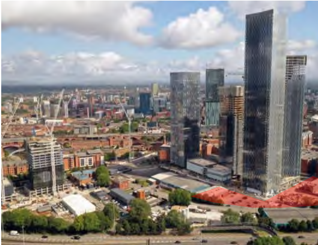
Figure 30: An aerial view looking north across the Site (shaded red) in 2019, illustrating the ongoing construction of the Crown Street development (left) and Deansgate Square development (right). The location of the Site is shaded red.
