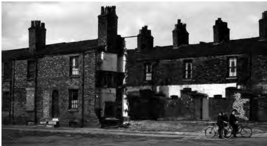
Figure 10: A view of the rear of houses on River Place (right) and houses fronting Alpha Street (left) during demolition in 1955. (Source: Manchester Archives)
