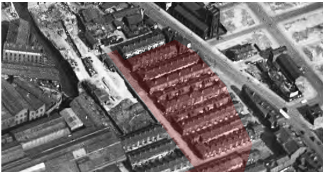
Figure 8: Looking east over the Site (shaded red) in 1939, showing the fine-grain nature of the residential terraced blocks. Note the beginning of slum clearances to the right of the image (Source: Britain from above).
