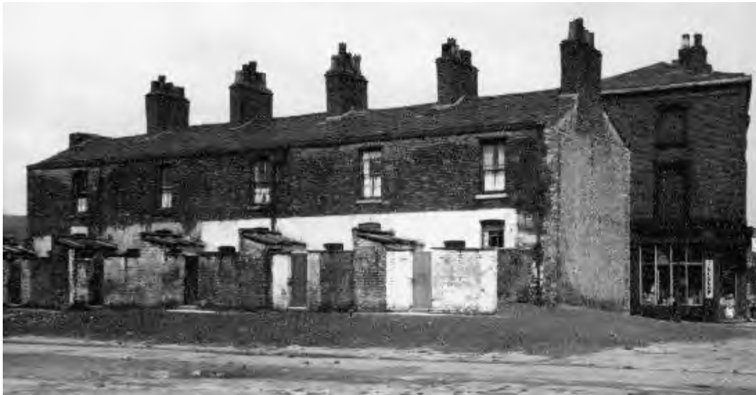
Figure 9: Alpha Street in 1955 showing its partial demolition. (Source: Manchester Archives)
