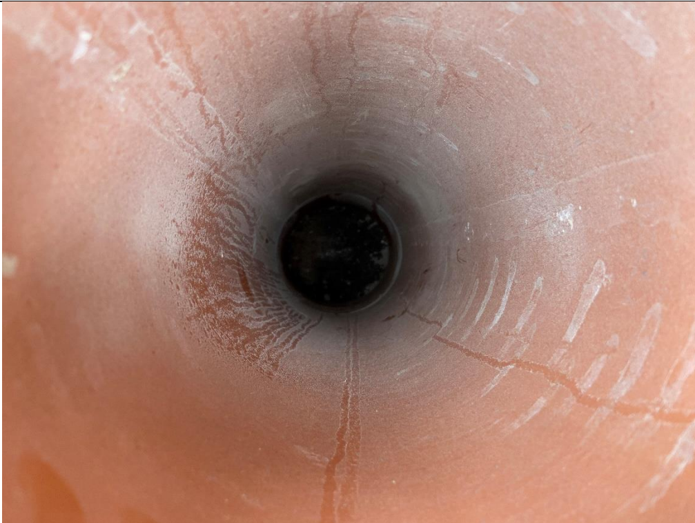
Photograph 3: Validation of Geotextile Membrane
