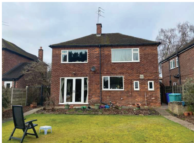
f) Existing rear facade
