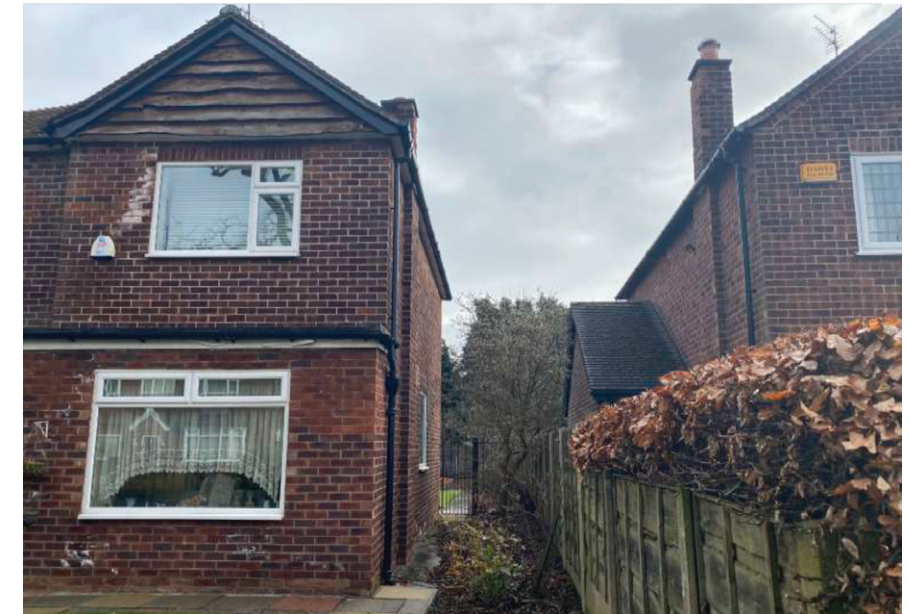
e) Existing sideway (south)
