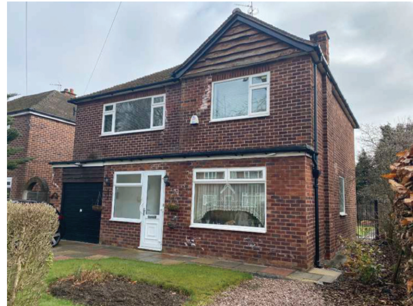
d) Existing front facade
