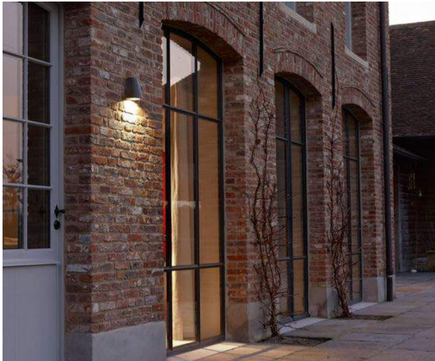
Reclaimed Brickwork, Shallow Brick Arches, and Crittall Style Window & Door Examples
