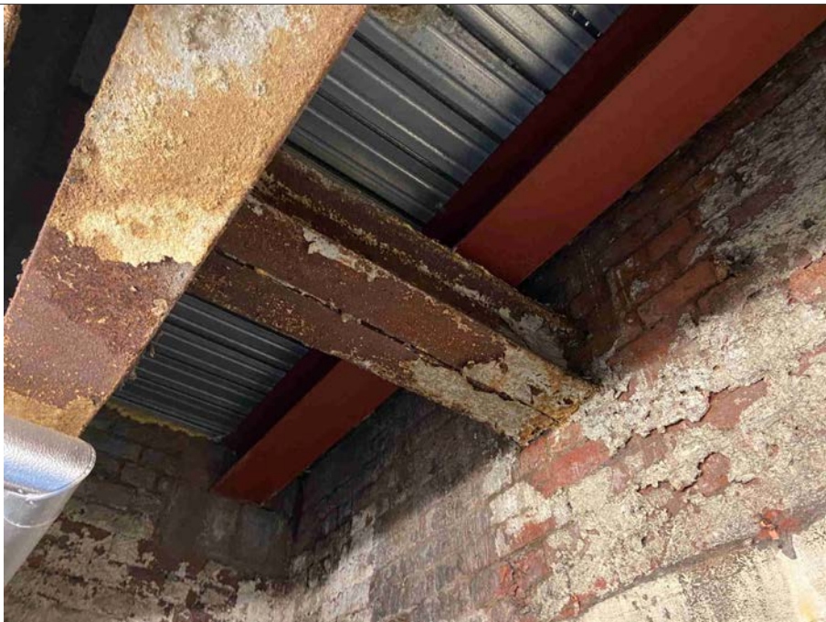
34: Basement boiler room soffit – note new steelwork and metal deck supporting car lift with original steelwork below
