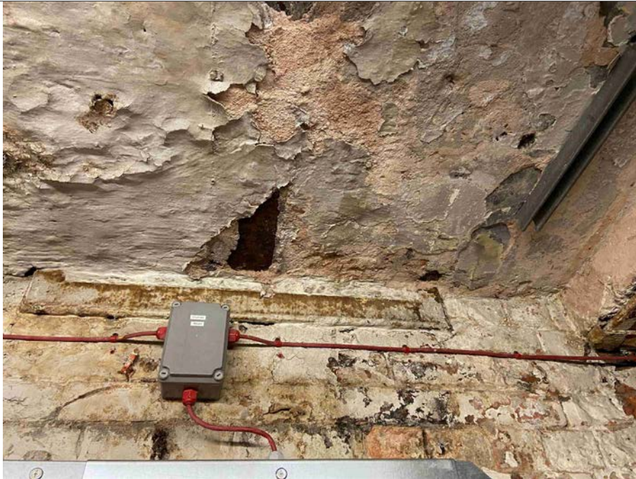
33: Basement boiler room soffit
