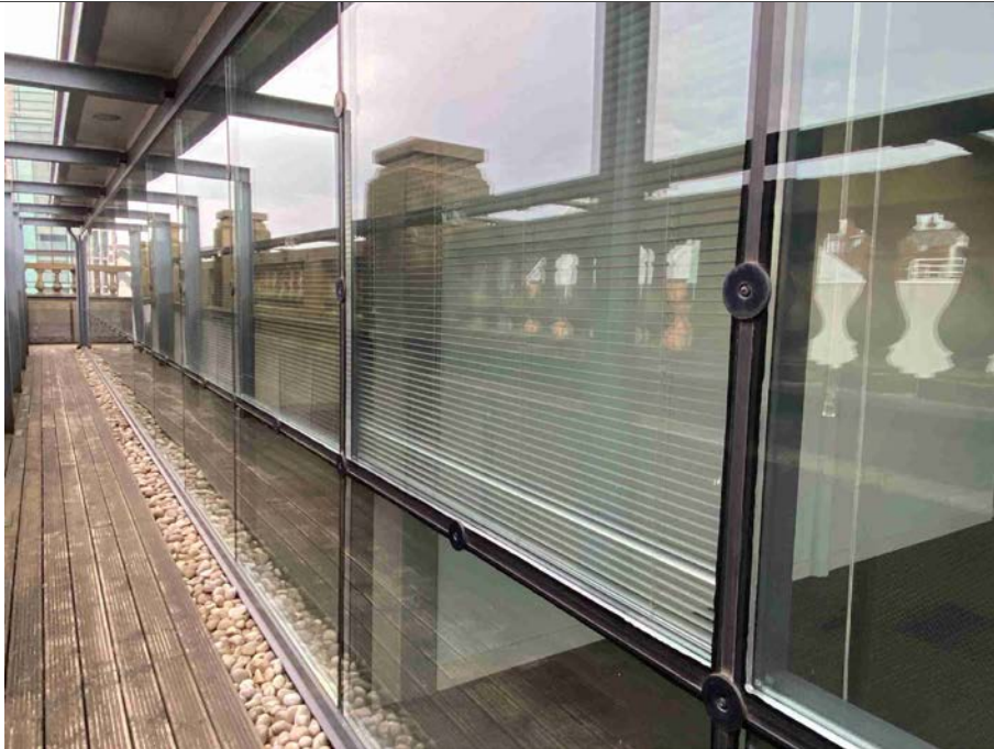
29: Face sealed curtain glazing to fifth floor office
