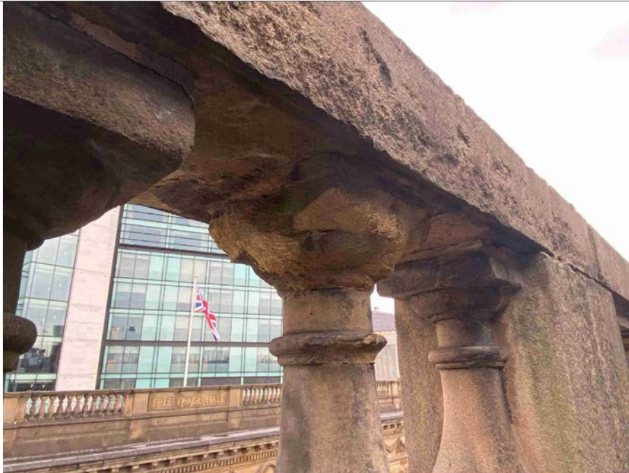
25: Example condition of stonework to balustrade
