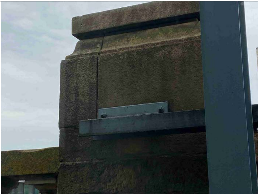
22: Example steel restraint tie to Peter Street and Southmill Street parapet stonework
