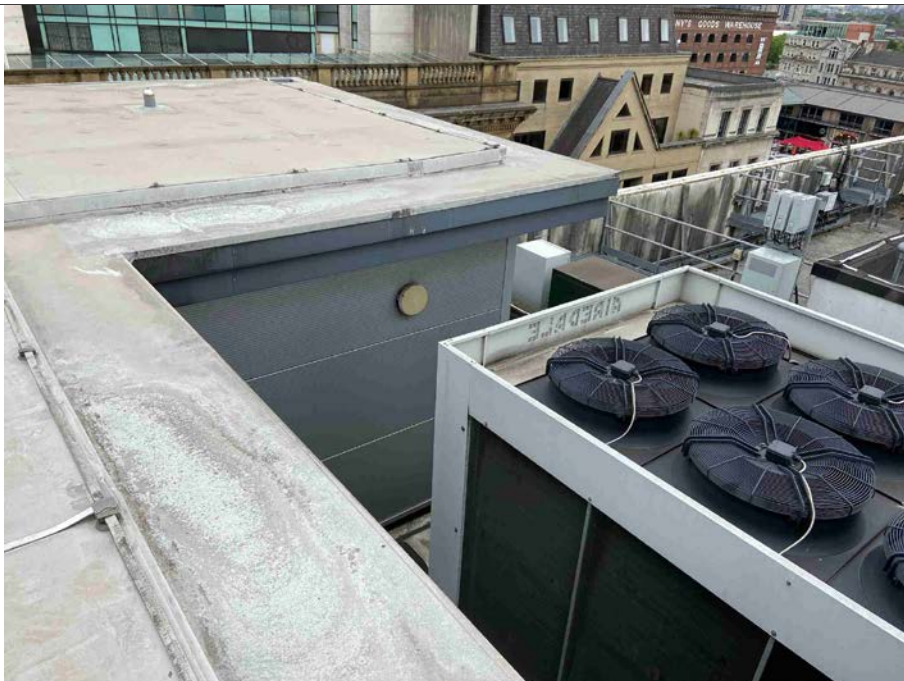
18: Main flat roof and central chiller plant (note composite panels)
