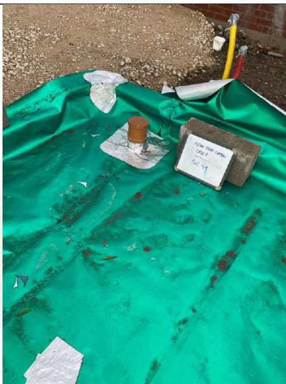
Photograph 6: Validation of Gas Membrane Installation
