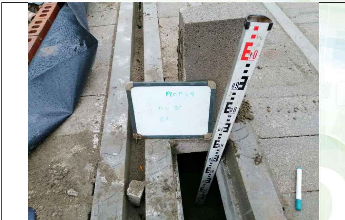
Photograph 4: Validation of Sub-Floor Void Space (min 150 mm)
