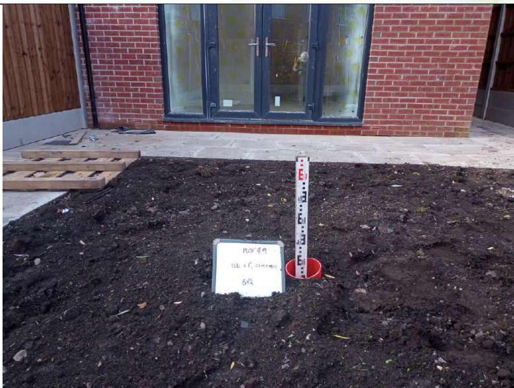
Photograph 2: Validation of Garden Capping Thickness
