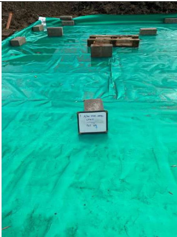
Photograph 5: Validation of Gas Membrane Installation
