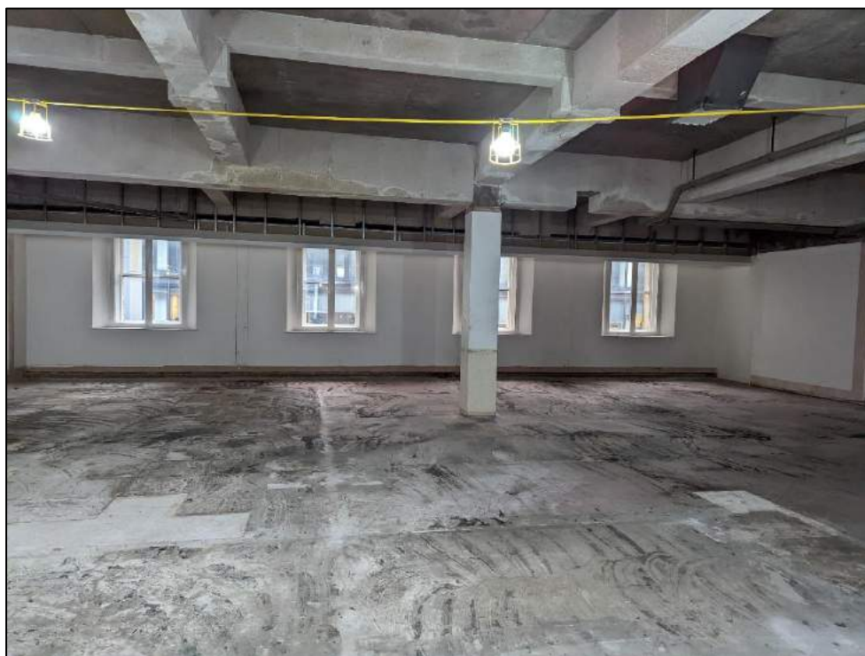
Plate 78: Room to southeast corner of extension
