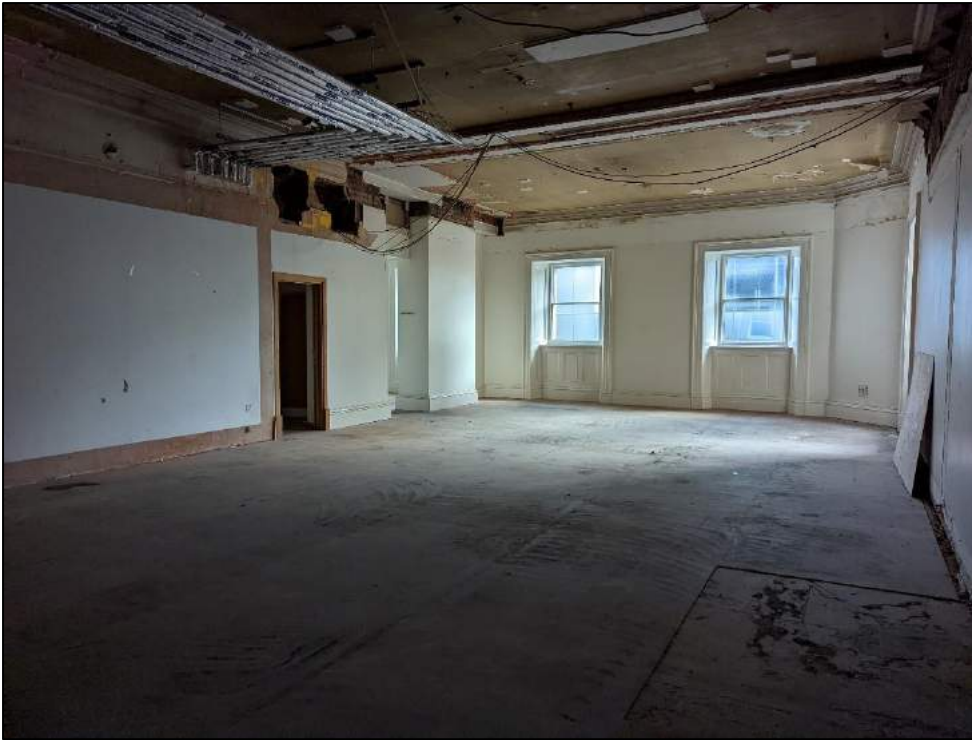
Plate 82: Room to southeast corner of original building
