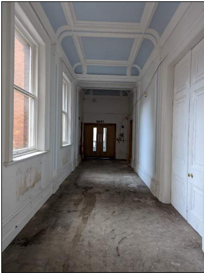
Plate 70: General shot of corridor looking north
