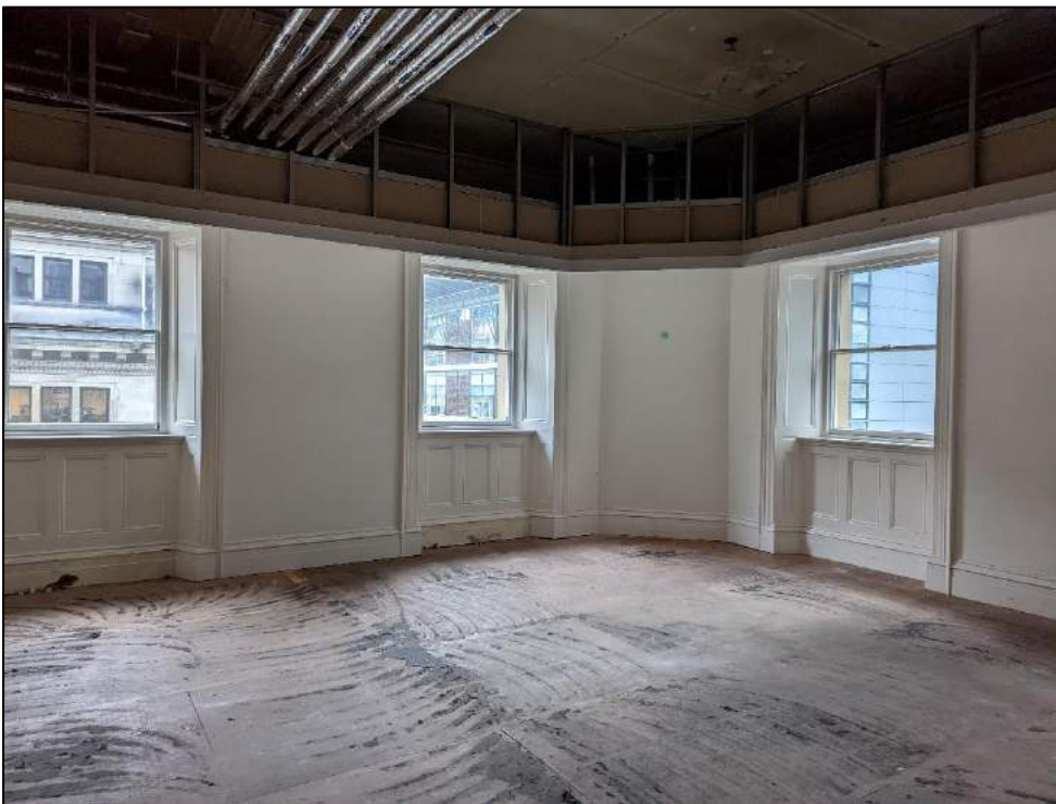
Plate 89: Large open space to north side of original building
