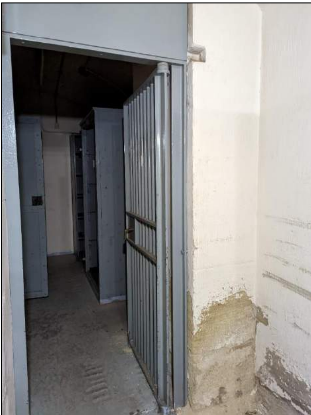
Plate 105: As above showing vault door
