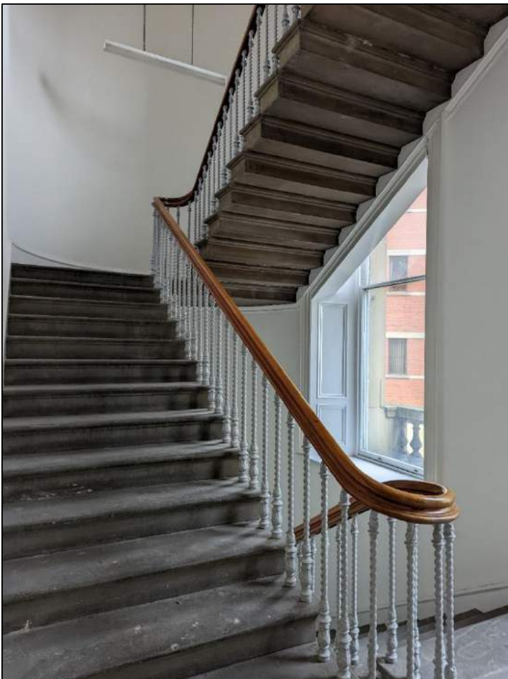
Plate 67: Staircase at northwest corner of building
