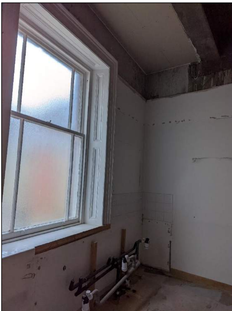
Plate 97: Stripped out WC in southwest corner of original building
