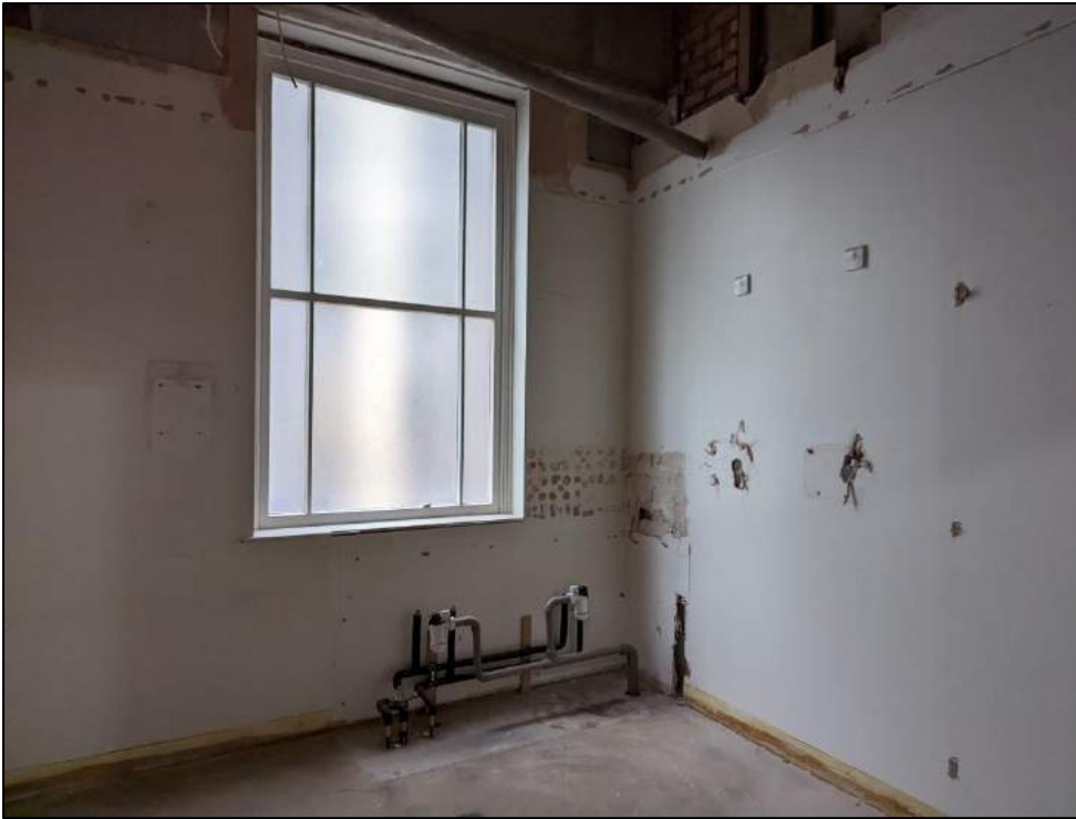
Plate 76: Room to northwest corner of extension
