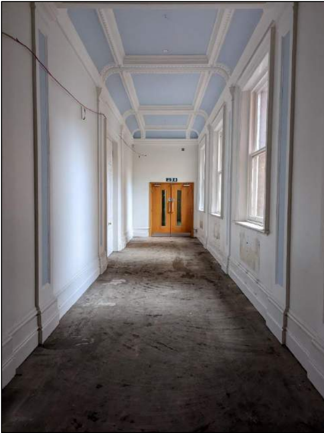
Plate 68: Western corridor linking office rooms
