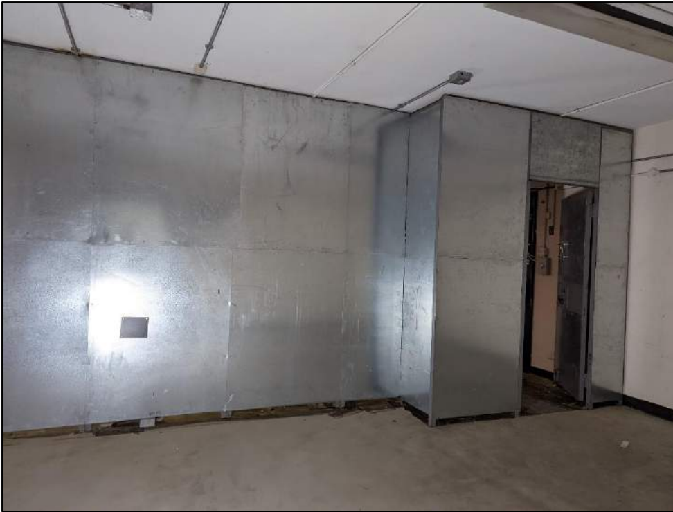
Plate 108: Central room of original building showing inserted wall and plasterboard ceiling
