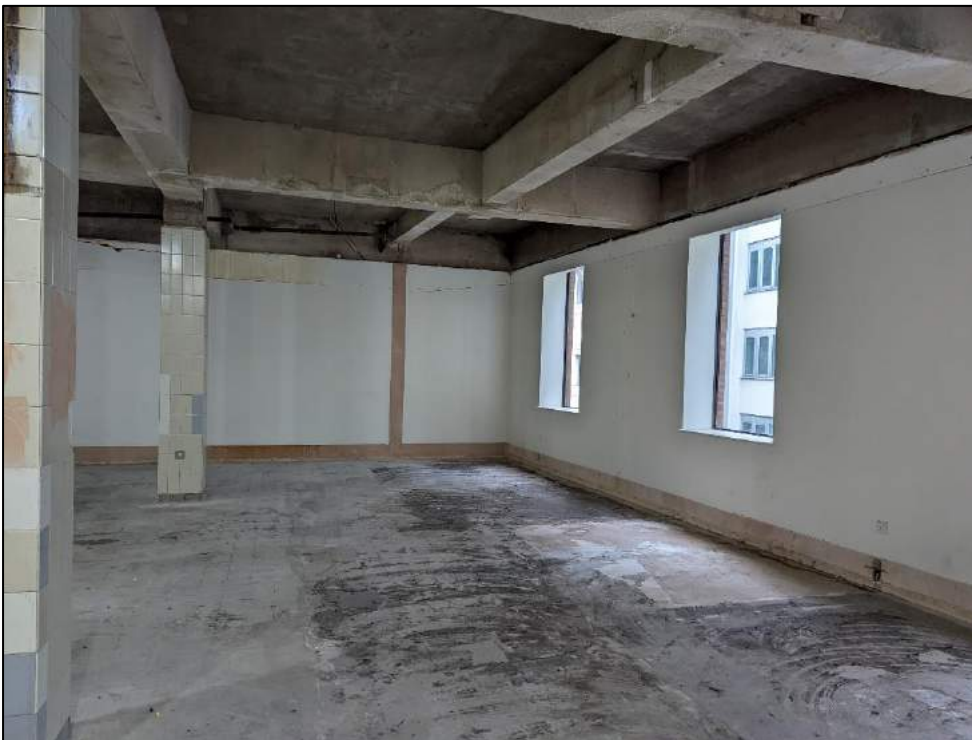
Plate 77: Room to southwest corner of extension
