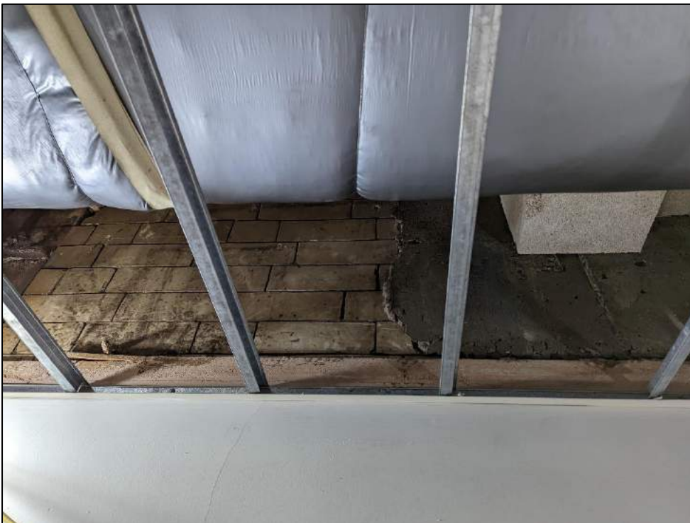
Plate 113: Detail of glazed bricks
