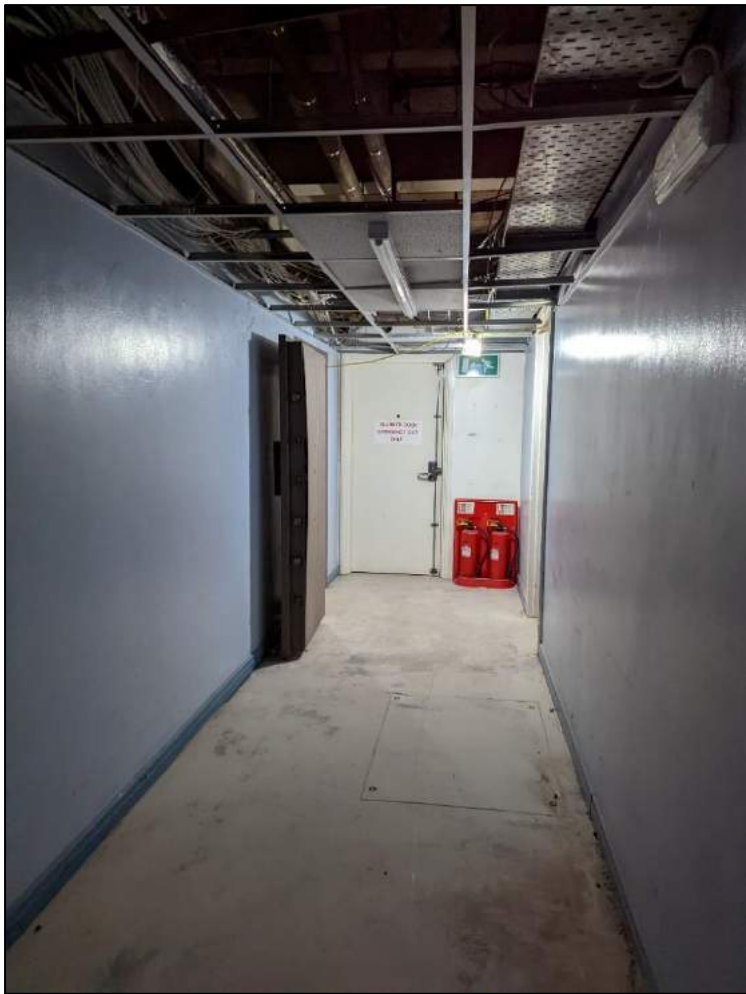
Plate 114: Corridor to west end of extension
