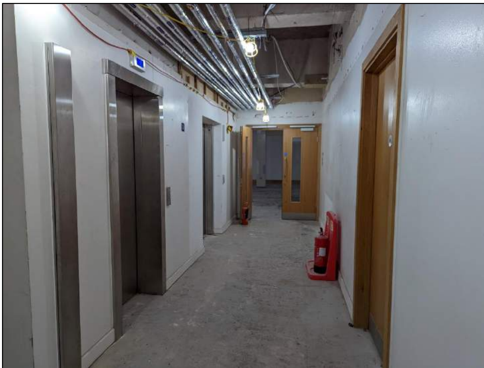
Plate 75: Inserted lift bank to extension
