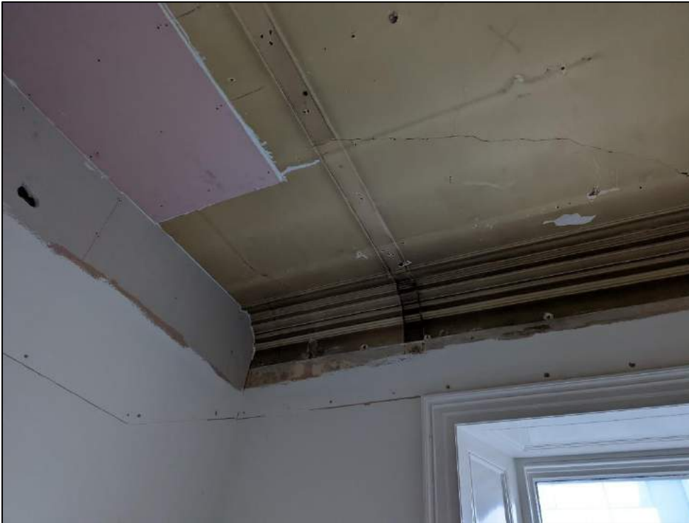
Plate 88: Ceiling detail of inserted office, showing cornice
