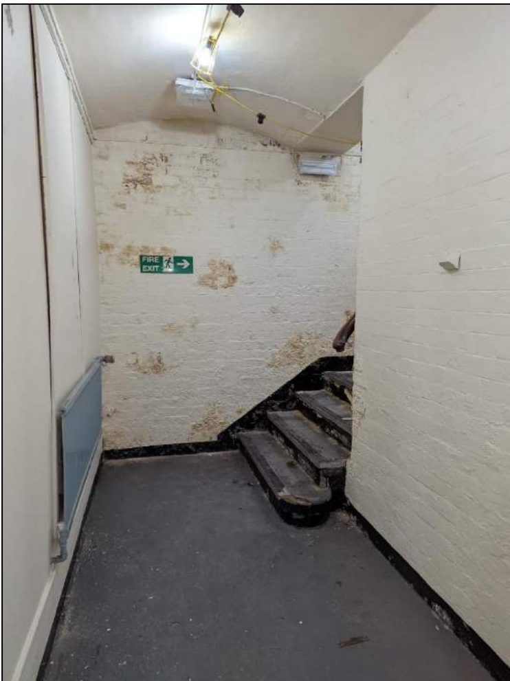
Plate 103: Staircase in northwest corner
