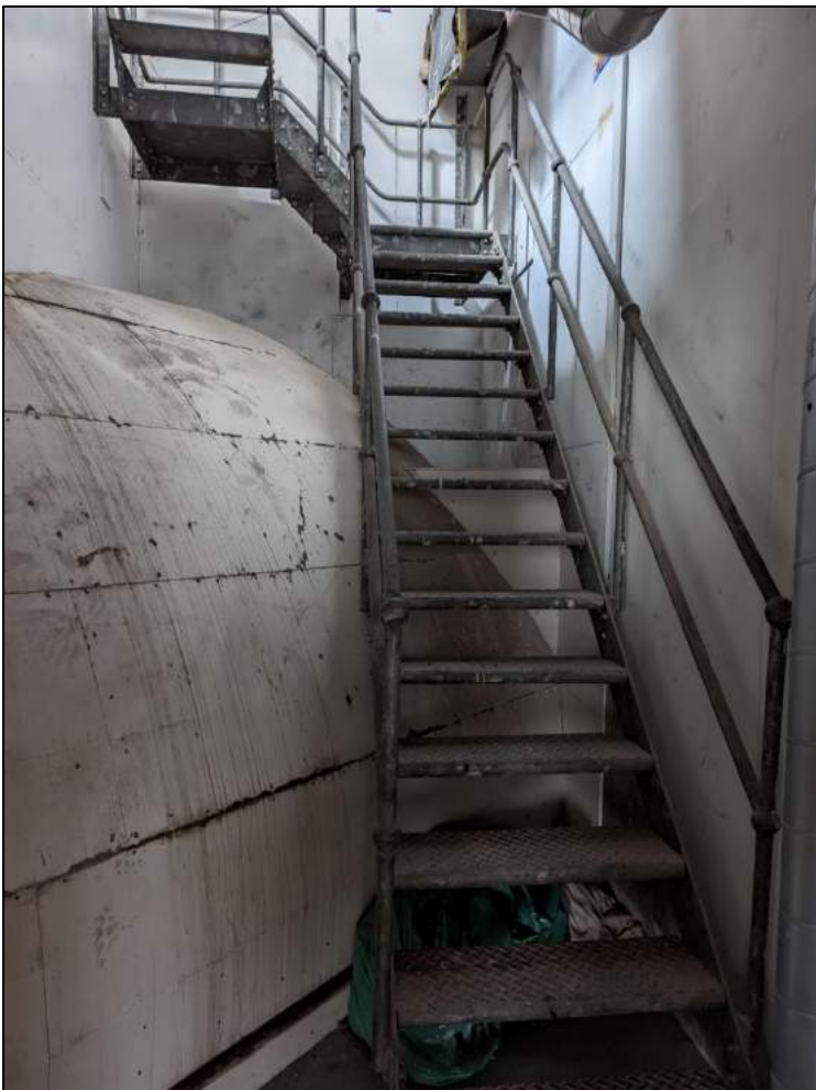
Plate 93: Metal staircase to roof access
