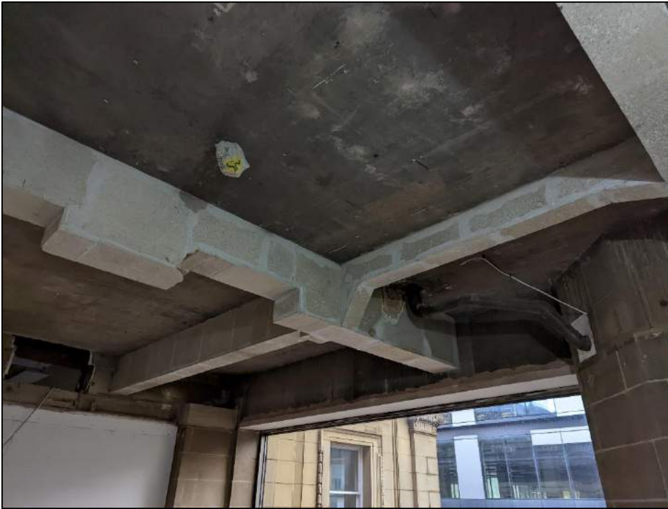
Plate 80: Detail of concrete ceiling construction
