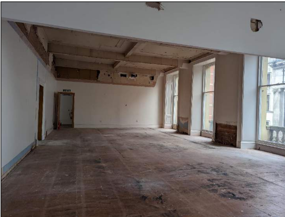
Plate 63: Northern room of original building
