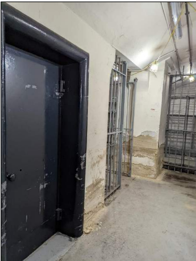
Plate 107 as above showing arched ceiling
