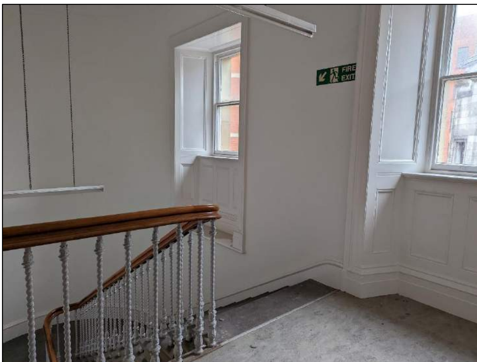
Plate 95: Staircase in northwest corner
