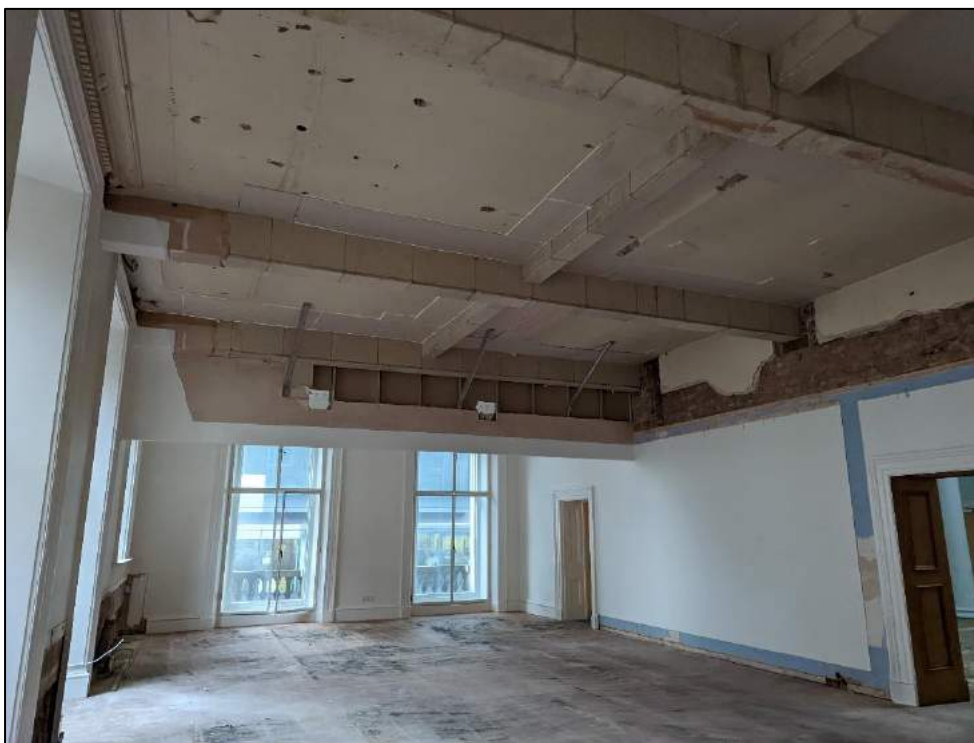
Plate 65: General shot of room
