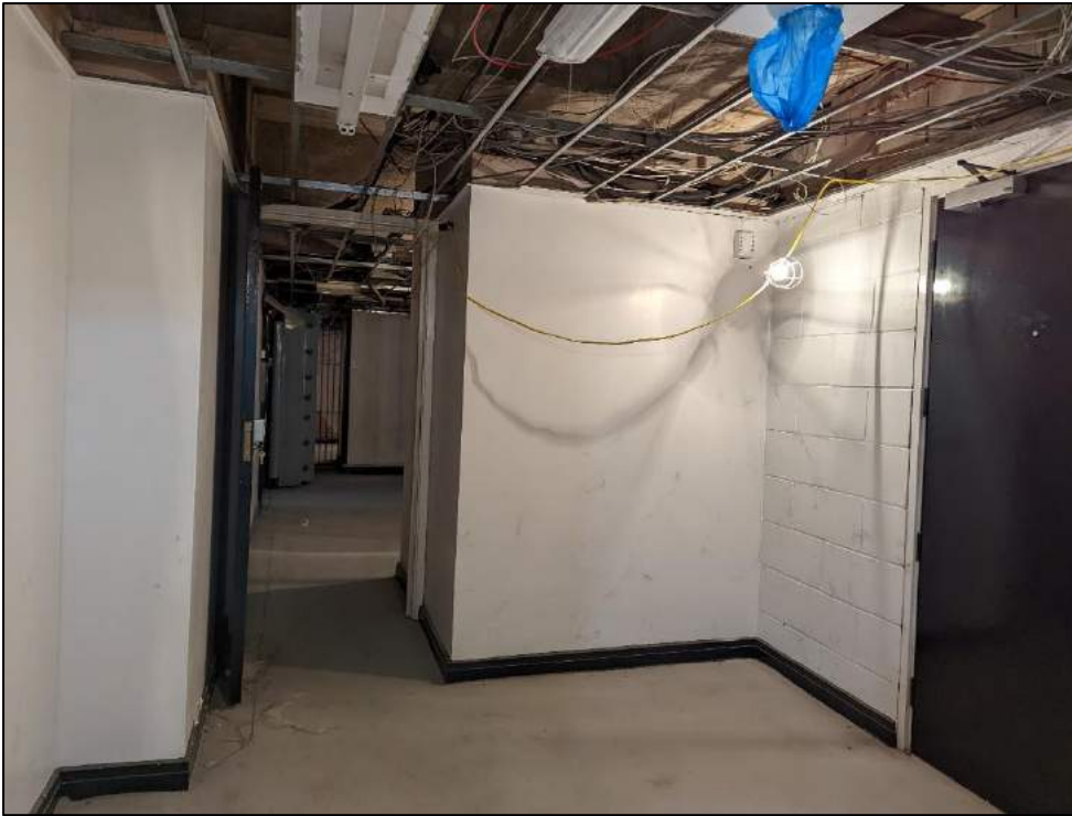
Plate 102: Northern vault area of original building
