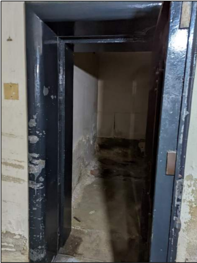
Plate 106: Further vault door
