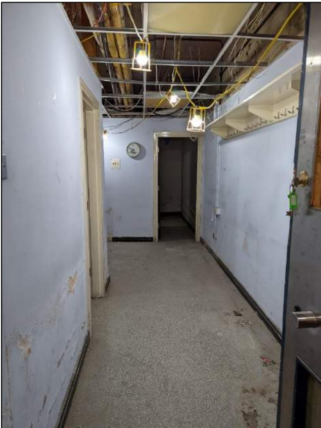
Plate 99: Corridor into rooms below arched wall area
