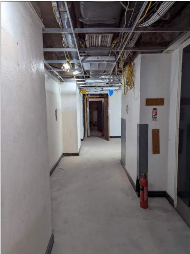
Plate 101: Corridor into vault area
