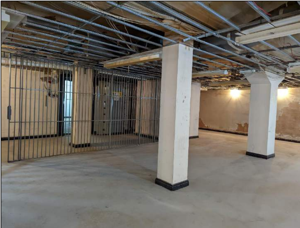
Plate 110: Southern room of original building
