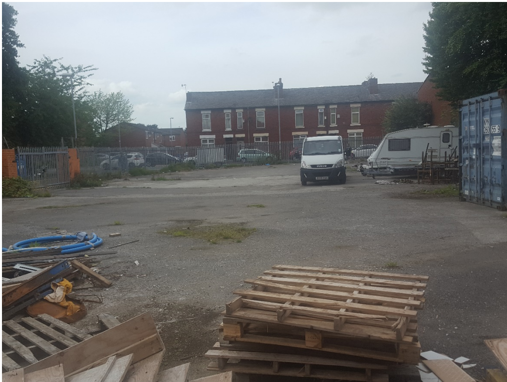
Figure 2 Overview of site, looking N
