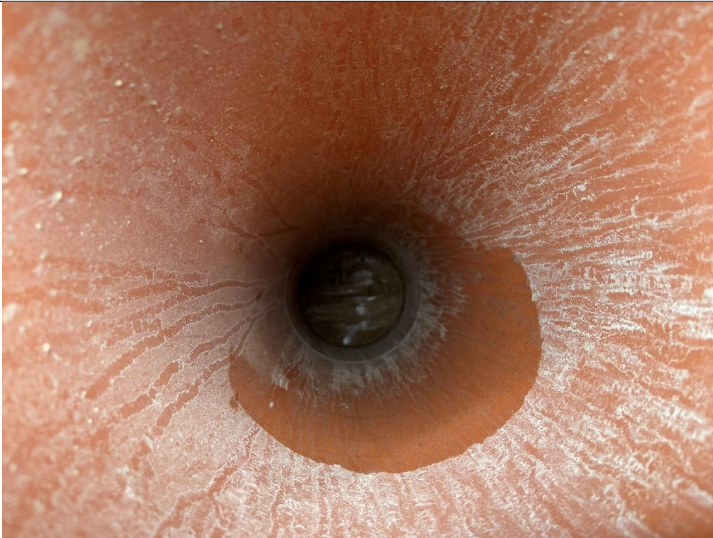
Photograph 3: Validation of Geotextile Membrane
