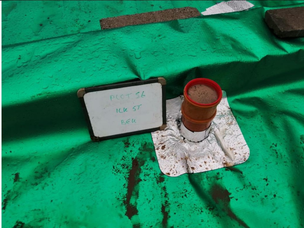
Photograph 5: Validation of Gas Membrane Installation
