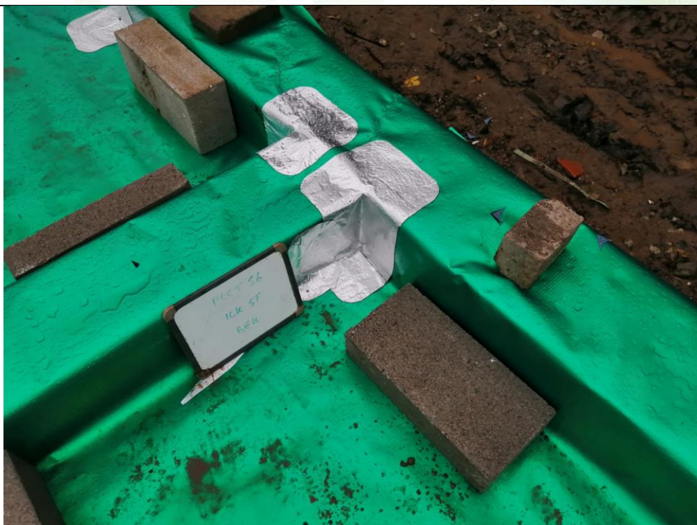
Photograph 8: Validation of Gas Membrane Installation
