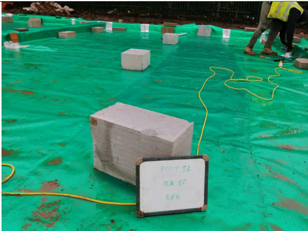
Photograph 6: Validation of Gas Membrane Installation
