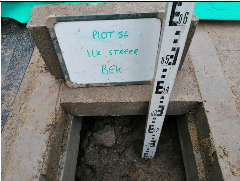
Photograph 4: Validation of Sub-Floor Void Space (min 150 mm)
