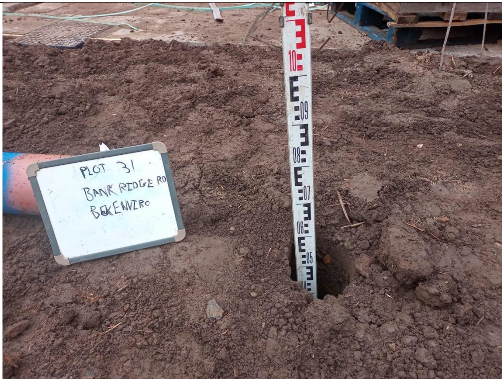
Photograph 1: Validation of Garden Capping Thickness
