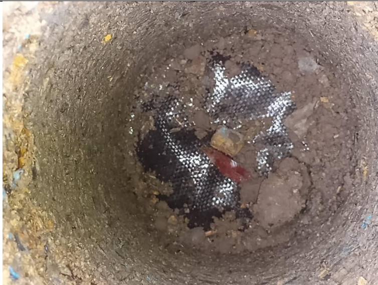
Photograph 3: Validation of Geotextile Membrane
