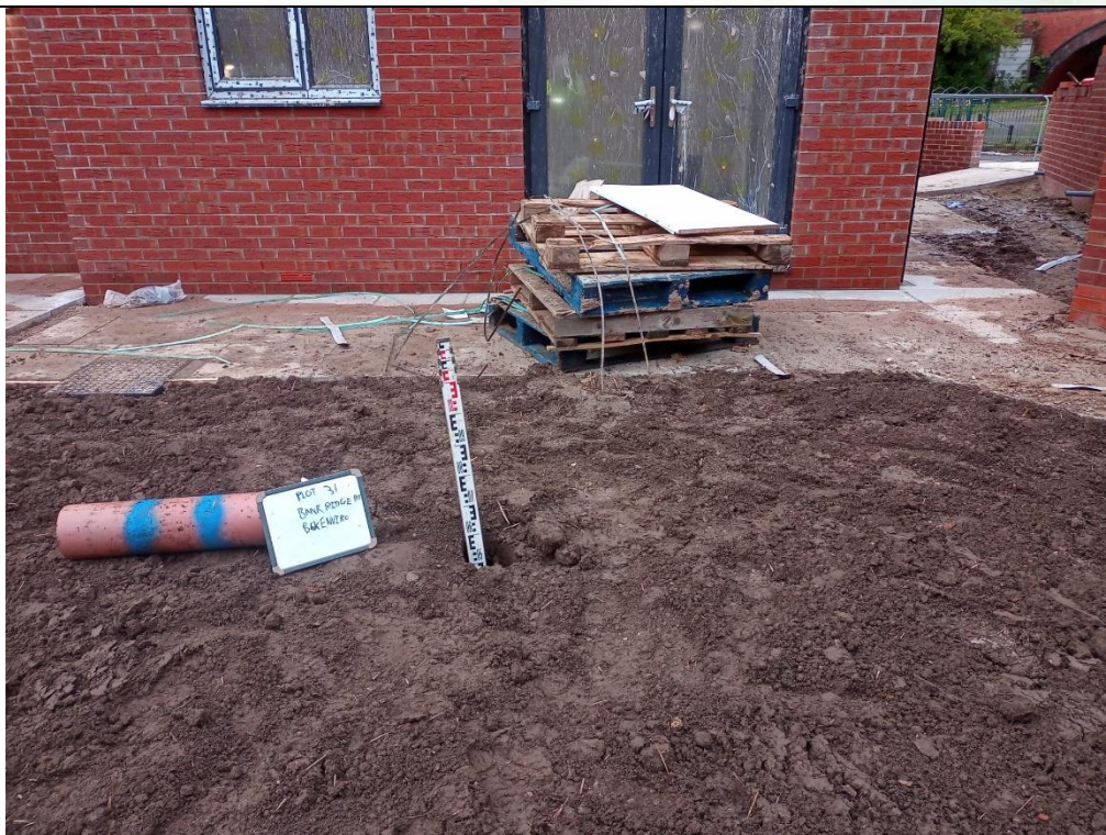
Photograph 2: Validation of Garden Capping Thickness
