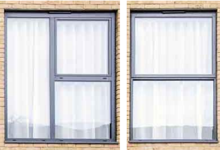
Aluminium casement windows, finish anodized dark grey
