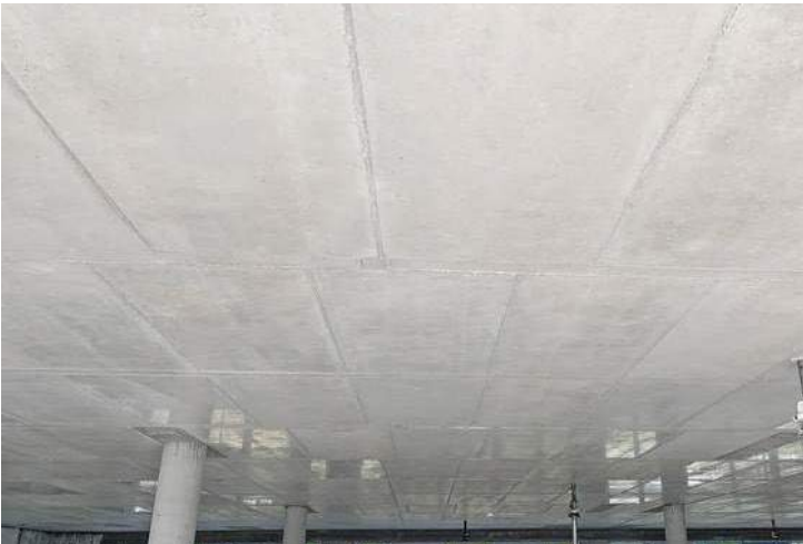
Internal exposed concrete soffit
