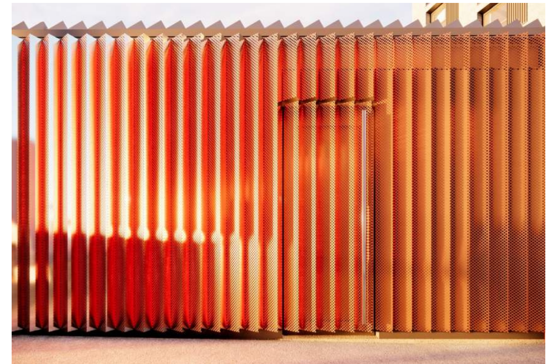
Detail of cabin triangle profile cladding
