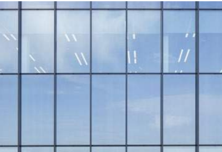
Aluminium capped curtain walling finish anodized dark grey
