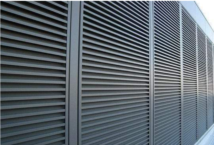
Louvre inserts to curtain walling, finish anodized dark grey
