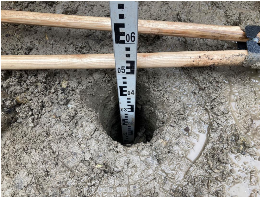
Photograph 3 VP02 showing 500mm of subsoil.
