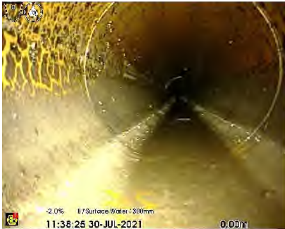
MH01 US LINE A_0-00m_113825.jpg, 00:00:19, 0.00 m Start node type, manhole, reference number: MH01, U.S LINE A
