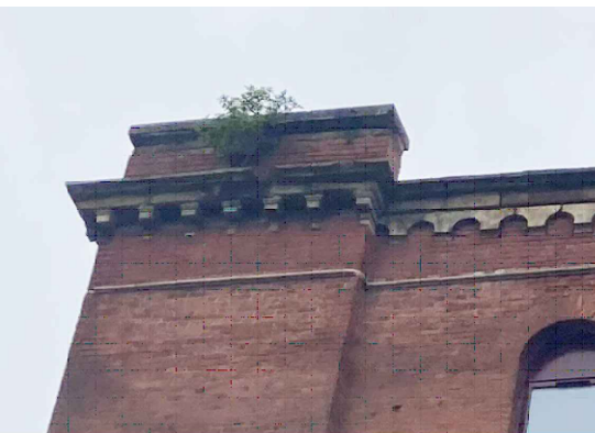
9. Crack between pier and main wall to be repaired with mortar to match existing.
