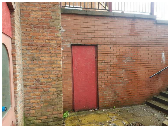
Existing basement door to be replace (extract from submitted Heritage Statement)
