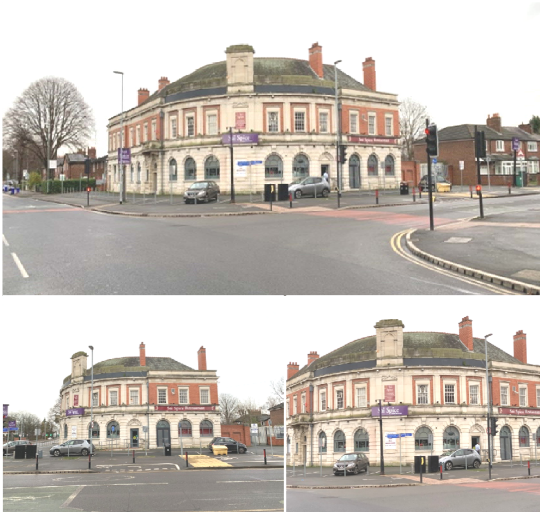
Fig 3.3 Present - Building Photographs
