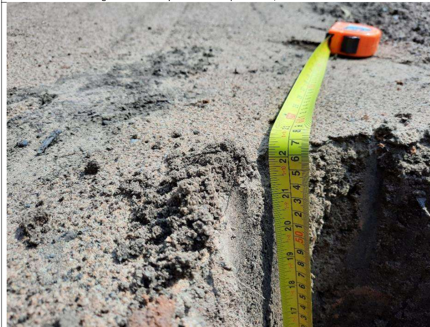
Plate 14: View showing depth of imported material at TS3/SS3.
