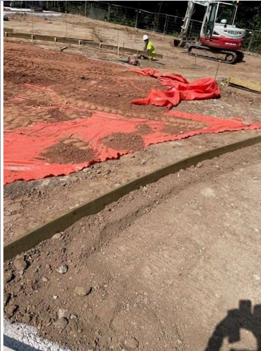
Plate 1: View showing the installation of the geotextile membrane beneath the landscaped areas.
