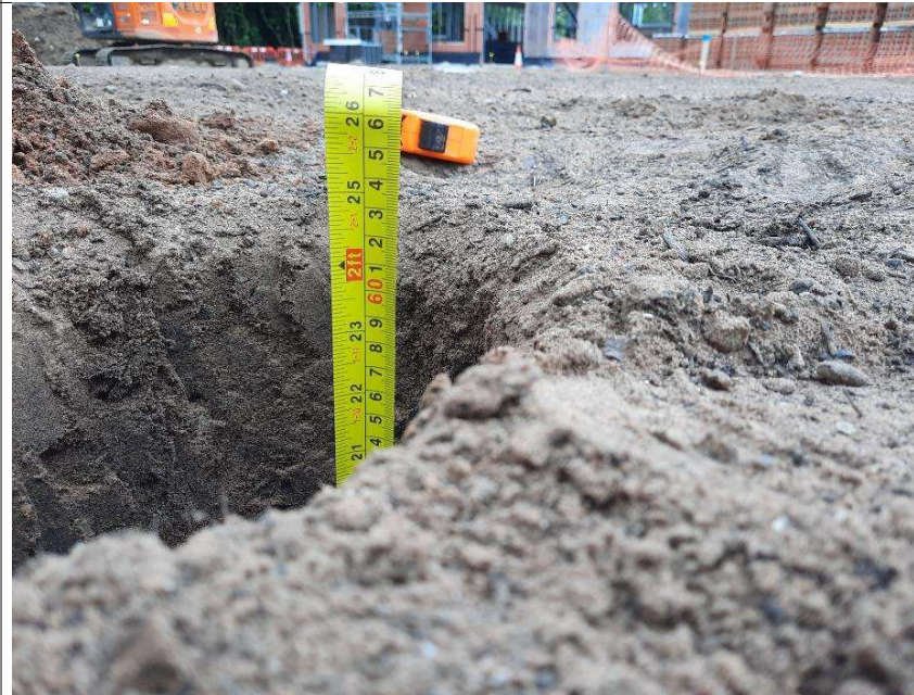
Plate 8: View showing depth of imported material at TS2/SS2.
