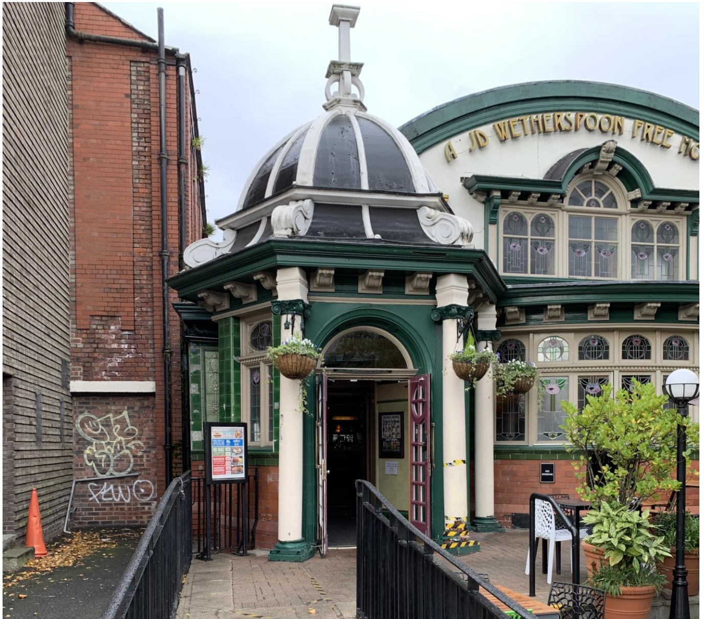
Photograph 1 The Sedge Lynn Entrance as seen from Manchester Road.
